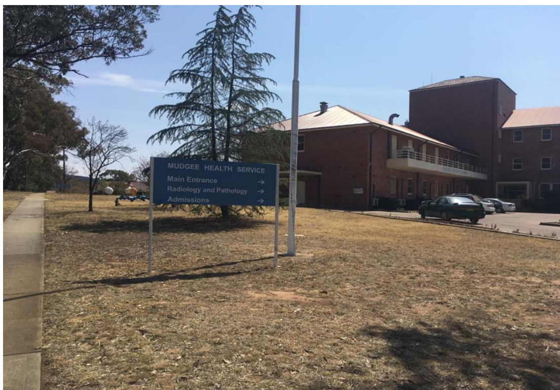
Photo 12 - Main Building from south-eastern corner of site looking west
