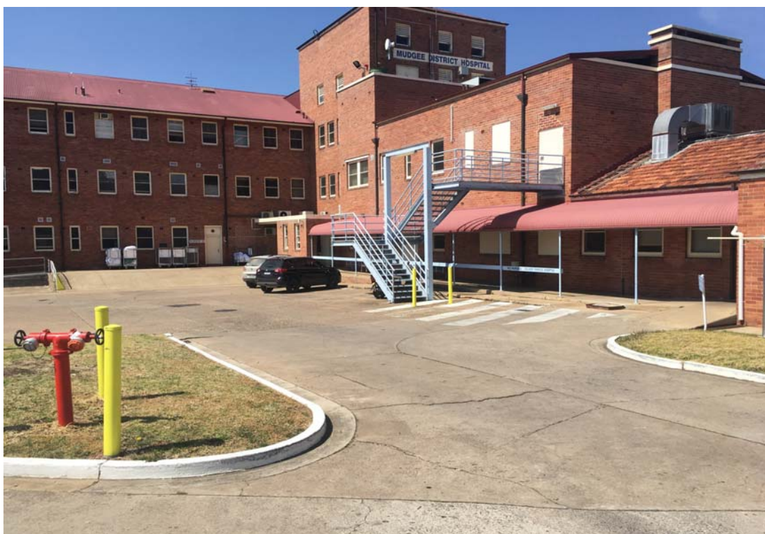
Photo 10 - North-western area of Main Building looking east
