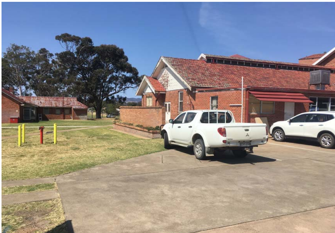
Photo 9 - Northern part of Boiler House looking east
