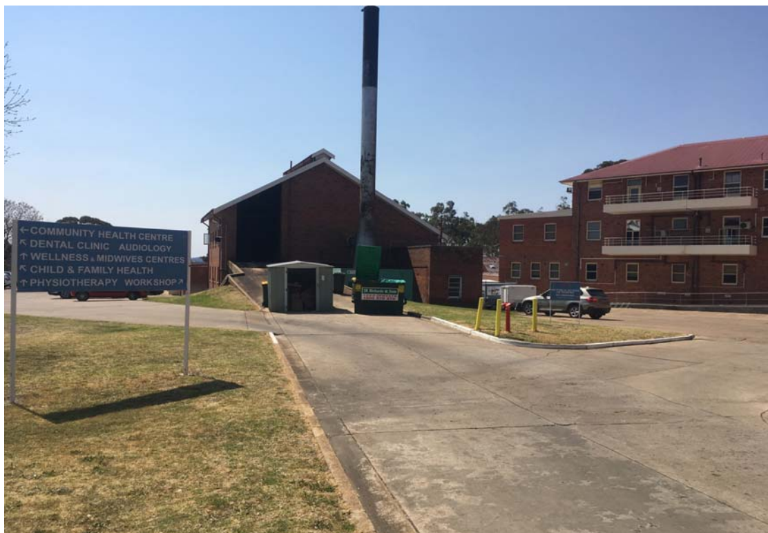
Photo 6 - View of Boiler House looking north
