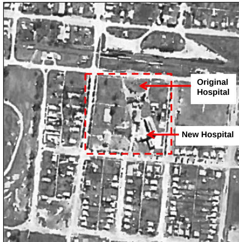
Figure 7: Aerial photograph of Mudgee Hospital, 1956
