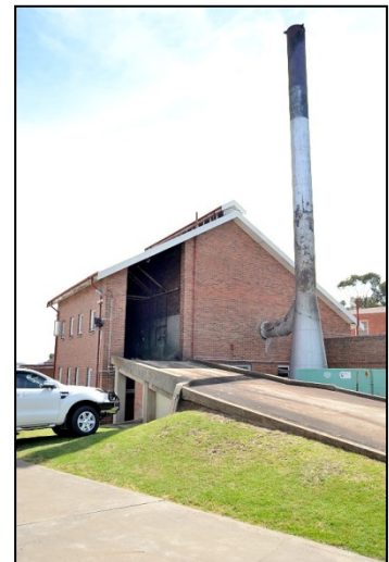
Figure 16: Boiler House and steel chimney
