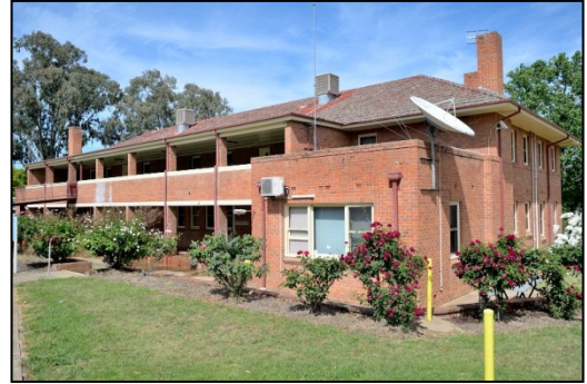
Figure 15: Community Health (northeast corner)
