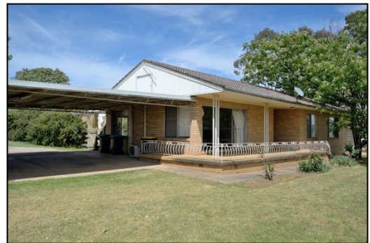
Figure 19: Residence - north view
