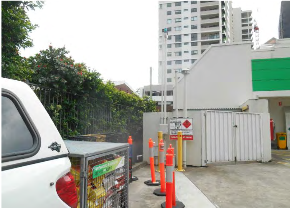
Photo 11 – Above ground liquid petroleum storage with ventilation directly adjacent to site boundary fence
