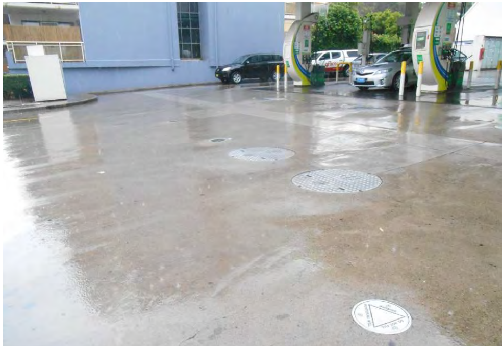
Photo 12 – Groundwater monitoring wells and underground storage tanks located at the service station
