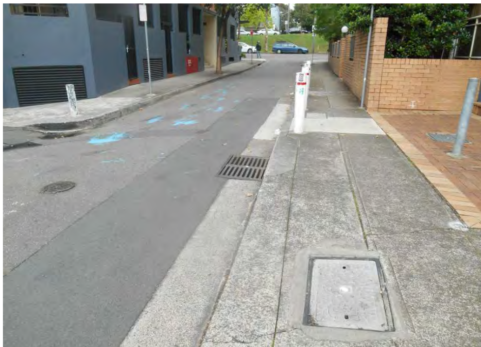
Photo 3 – Minor cracking along footpath and slight staining
