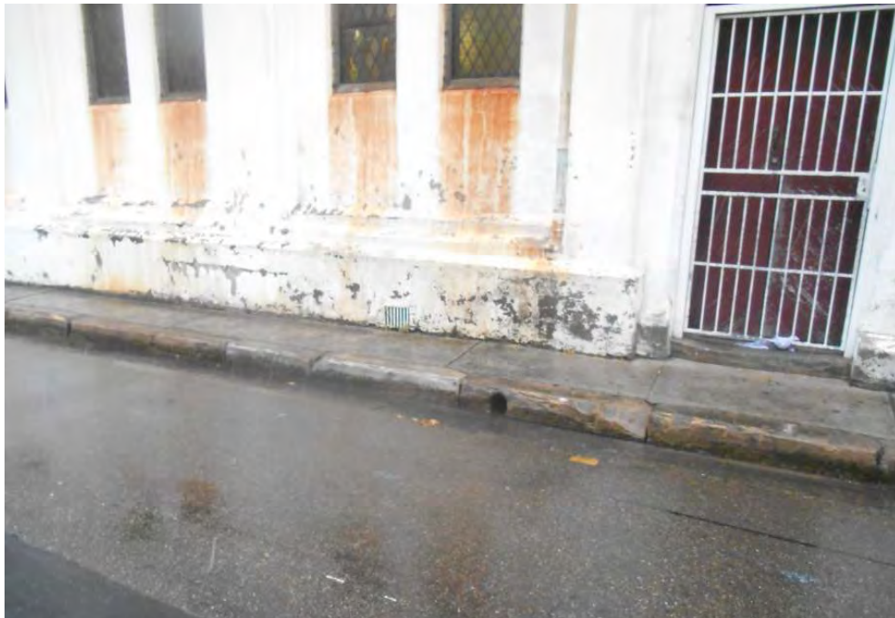
Photo 16 – Open drainage and ventilation for the church. Visible staining and degradation of the building and footpath
