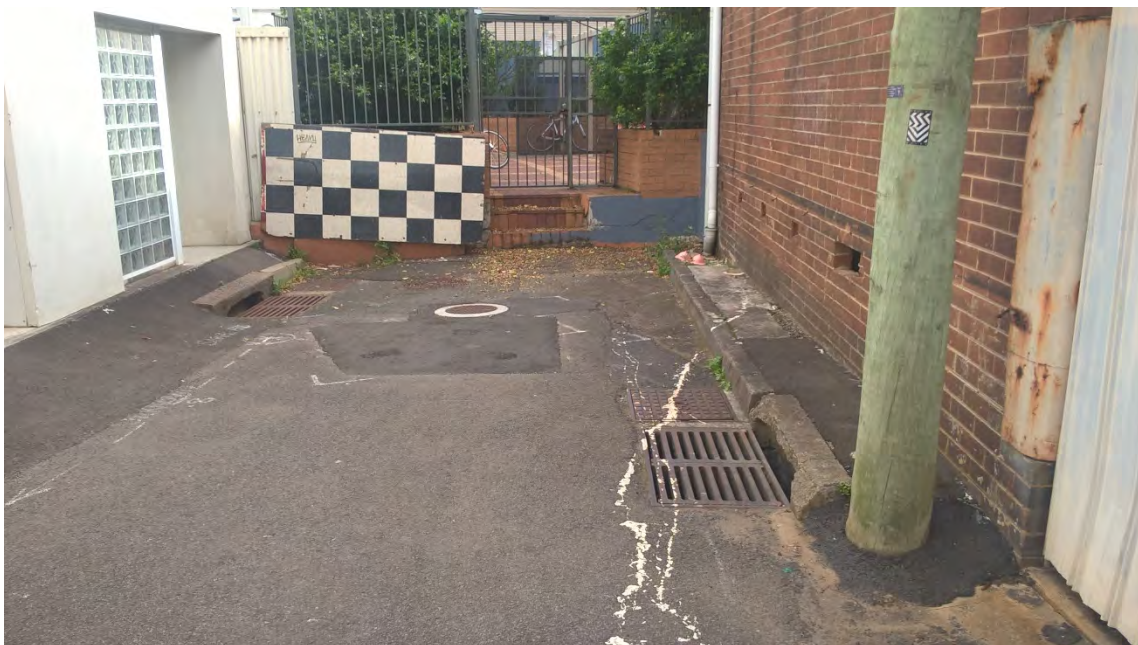
Photo showing existing courtyard is about 3 steps (600mm) higher than the street level with the lowest point at the left kerb inlet pit. The retaining wall behind the black and white chequered board have collapsed.
