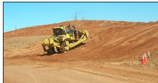
Photograph 10. Spreading of soil-rock mixture on the batter with a D9 dozer.
