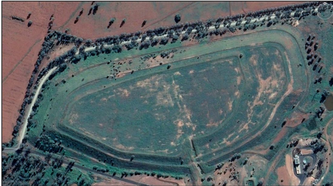
Photograph 4. The WRE at Peak Hill Gold Mine has a comparable benched design to the existing WRE's at Tomingley Gold Mine.
