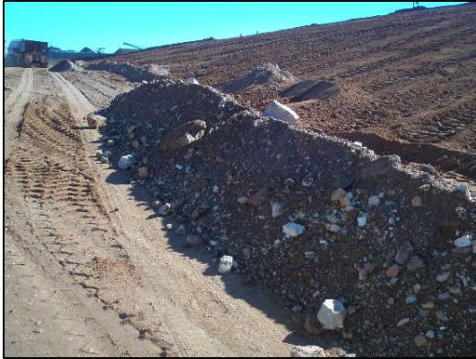
Photograph 7. Soil-rock mixture placed at the toe of the batter, prior to spreading.
