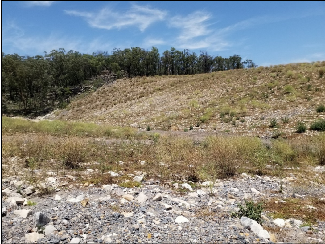
Photograph 12. Example of a batter with a high degree of surface roughness in the early stages of rehabilitation. Roughness was created by placing mixing rock with topsoil then pushing it down the batter. Location near Mudgee, NSW.
