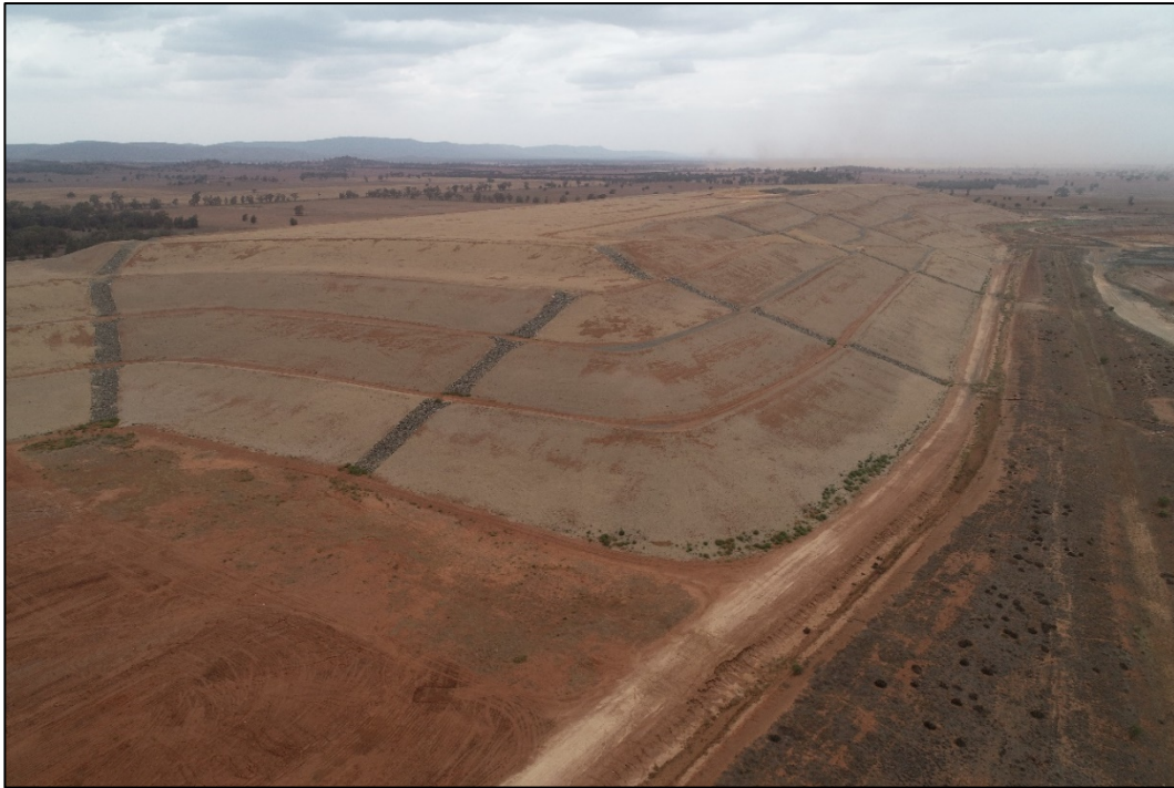
Photograph 1. Looking south-east at TGO's WRE #3. Benches drain laterally into the rock chutes then discharge at the toe of the WRE. This photography was captured after the WRE was hydromulched for revegetation circa December 2019 (Courtesy, the Applicant, May 2021).
