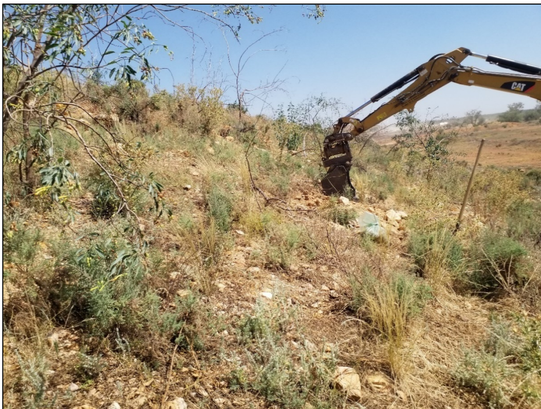
Photograph 11. Example of a rehabilitated batter with a high degree of surface roughness due to the appreciable rock content in the spoil materials that have been ripped along the contour. Location near Cobar, NSW.
