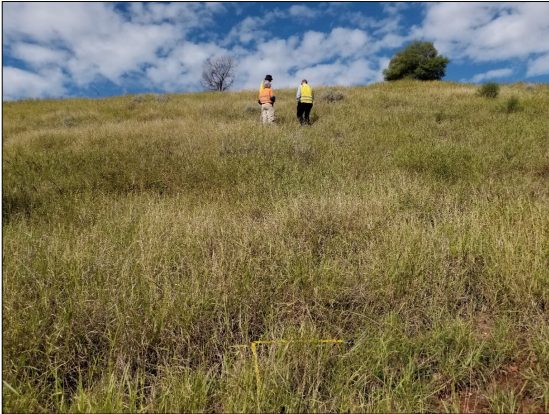
Photograph 5. Vigorous grass cover on the batter of the WRE at Peak Hill Gold Mine.
