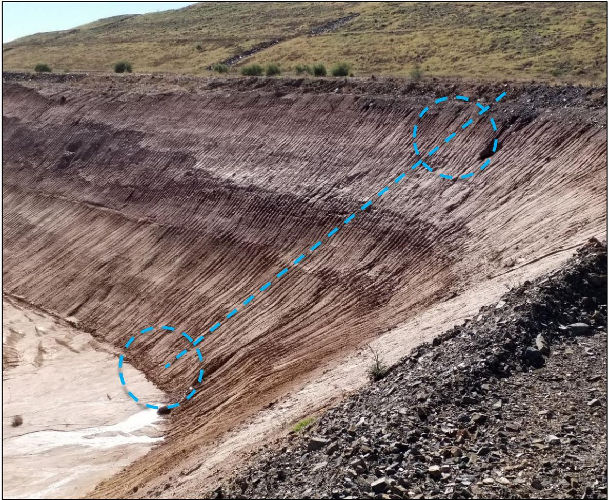
**Photograph 1.** Example of scarification on pit walls at TGO resulting from excavating with a toothed bucket. There is also an incidence of tunnel erosion on this batter, as indicated by the blue dashed line.
