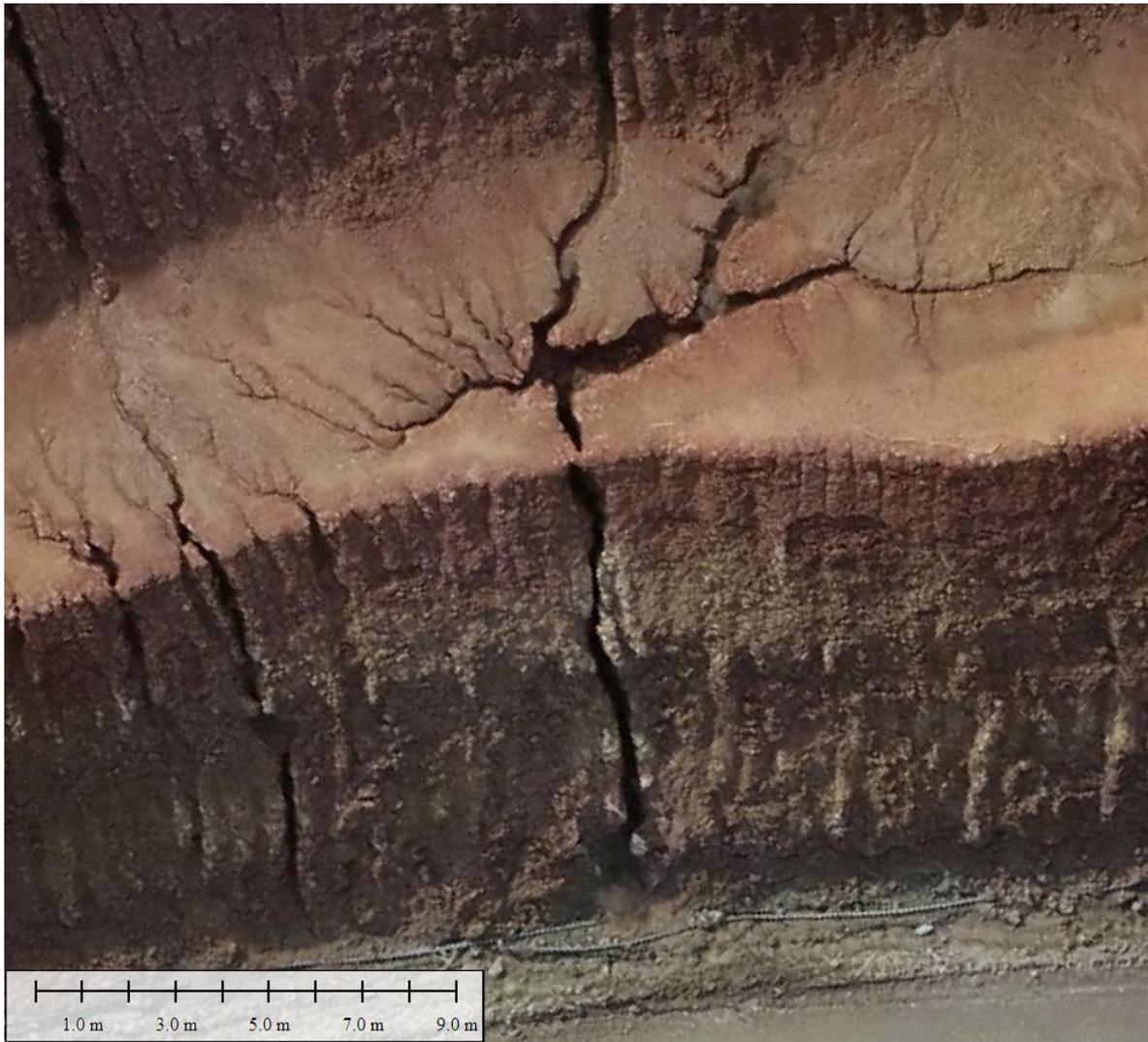
Photograph 2: Tunnel erosion in the berm batter sequence in Wyoming 1 Open Cut.
