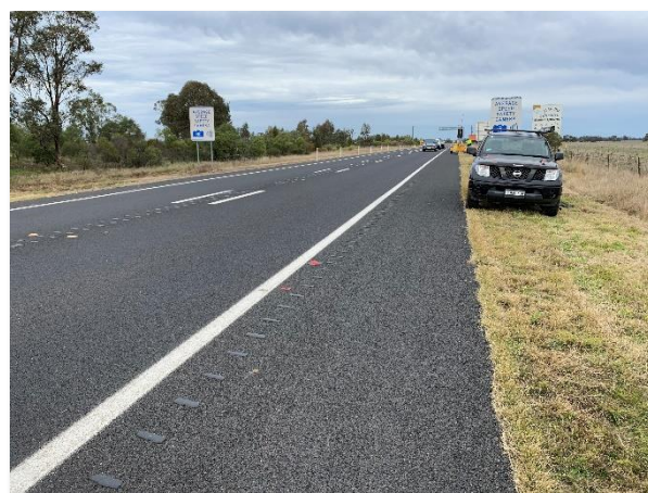
2. Newell Highway near TP7 looking south
