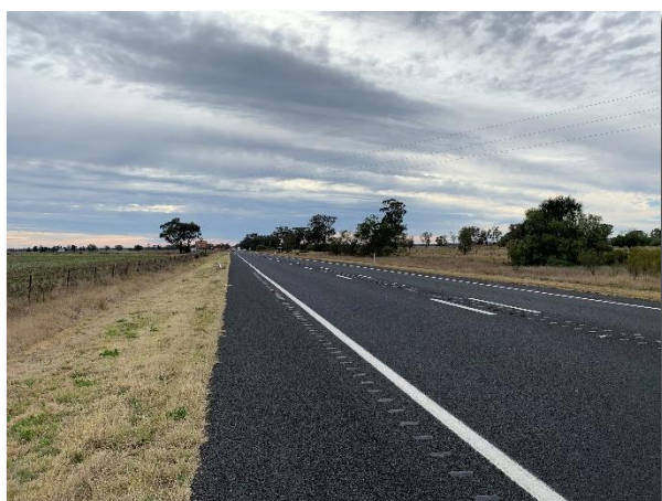
1. Newell Highway near TP7 looking north
