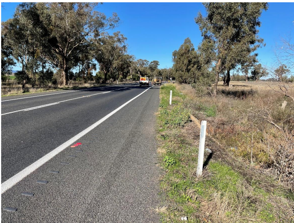
1. Newell Highway near TP27 looking south
