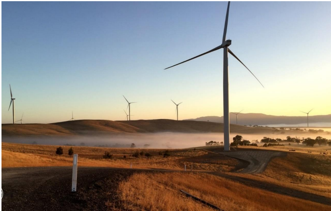
Photo 1 Wind Farm Post Construction 11
