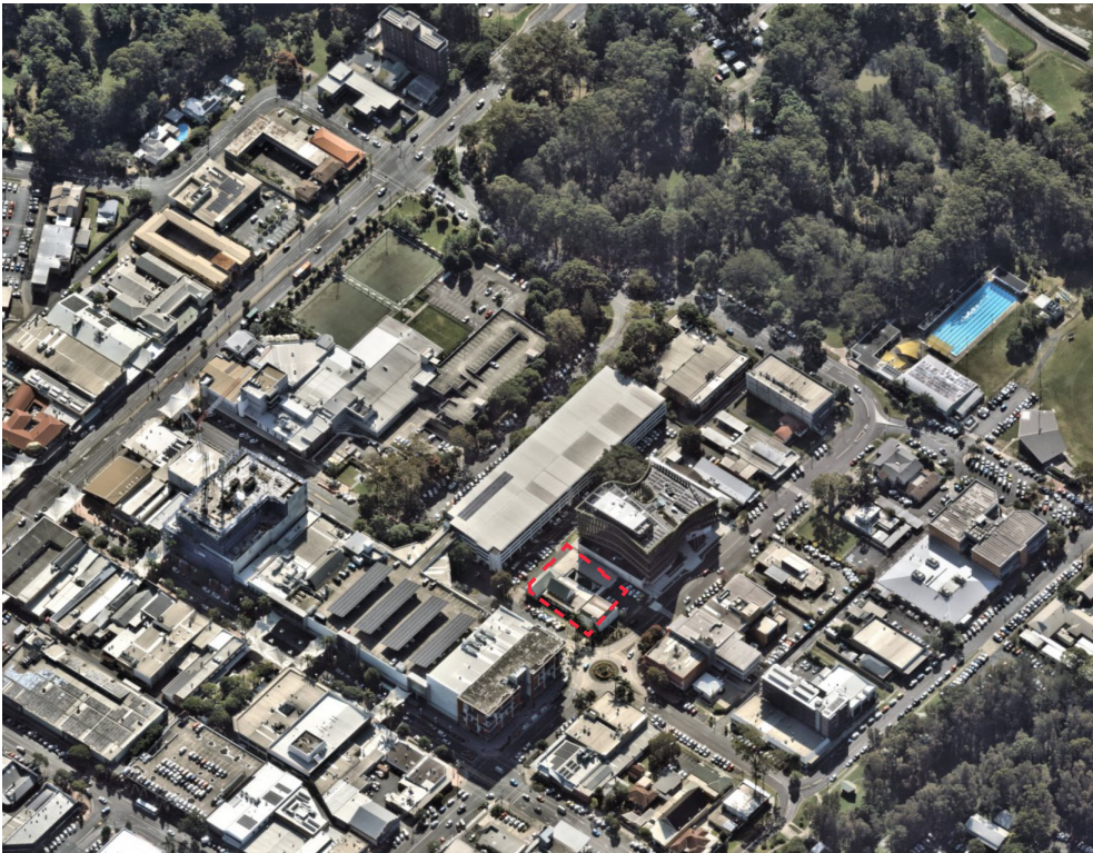
Above: The Project Site, located in the heart of the Coffs Harbour CBD.
