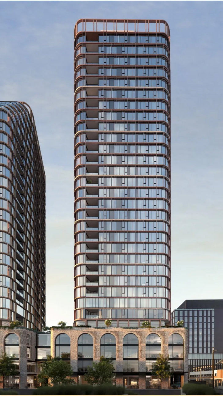
Above: The Store apartments, Newcastle NSW - 107m, Under Construction, Source DOMA
