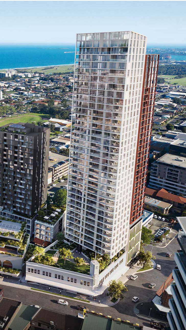
Above: WIN Grand Apartments, Woolongong NSW- 123m, approved for development. Source: Colony Six
