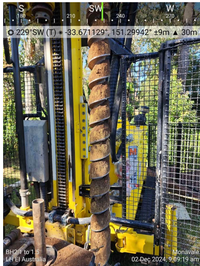
Photograph 11: View of soil material at BH2M during drilling (2/12/24)
