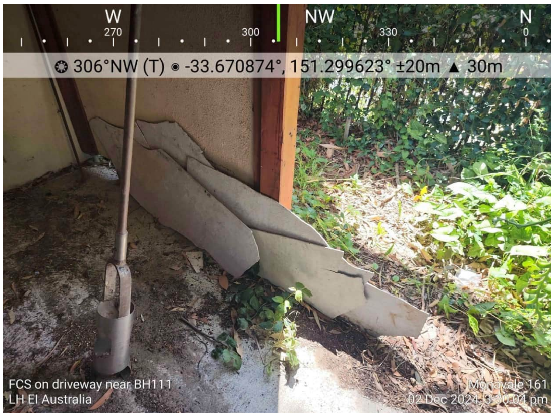
Photograph 3: Visual of Fibre Cement Sheetting located in garage of 161 Darley Street West (2/12/2024).
