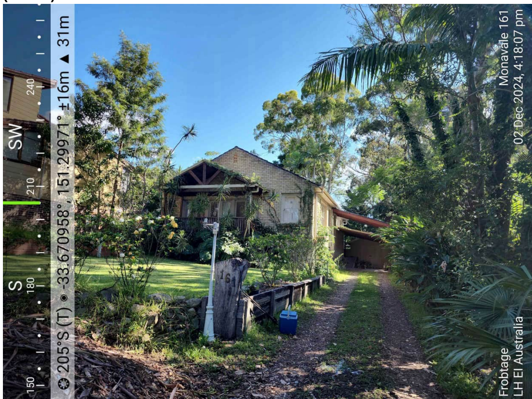
Photograph 8: View of frontage at 161 Darley Street West (2/12/24).
