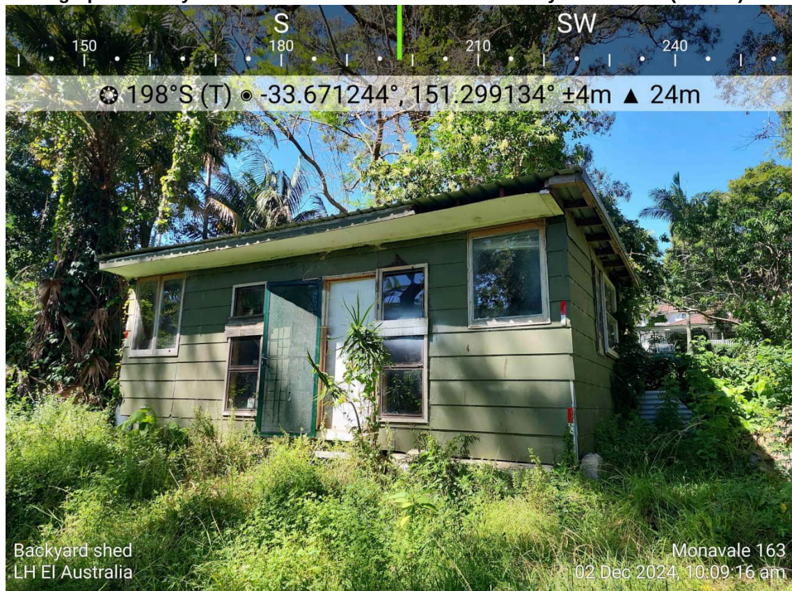
Photograph 6: Backyard shed located at 163-165 Darley Street West (2/12/24) .
