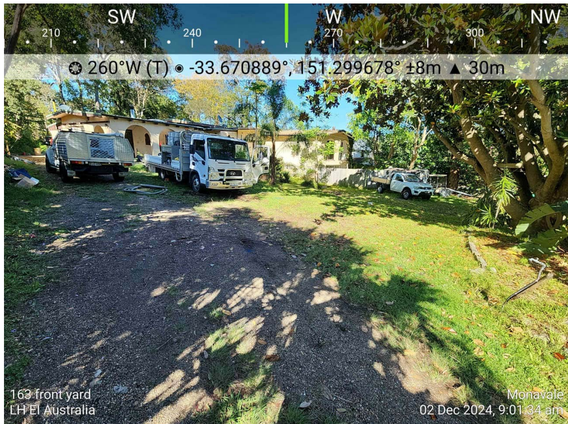
Photograph 1: Front view of 163-165 Darley Street West (2/12/2024).
