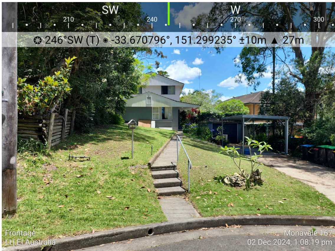
Photograph 9: View of frontage at 167 Darley Street West (2/12/24)
