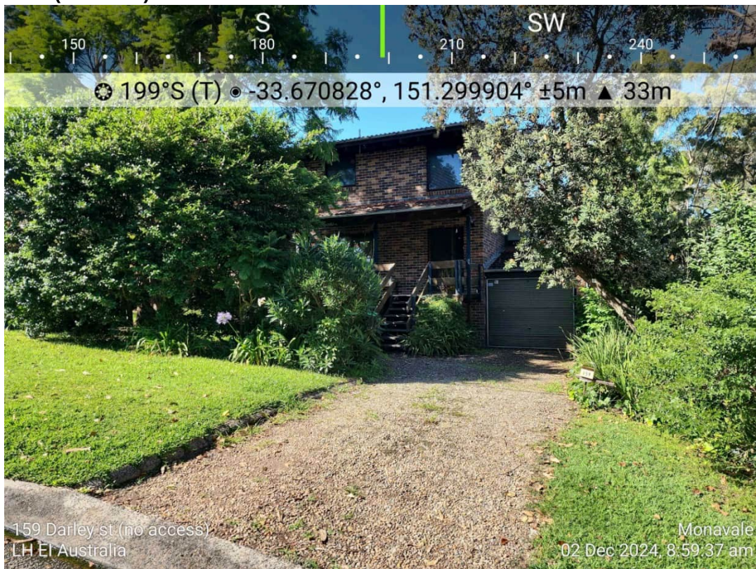
Photograph 4: Front view of 159 Darley Street West (2/12/2024).
