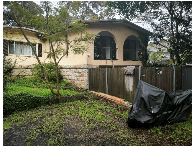
Figure 22 – 163 A Darley St front yard.
