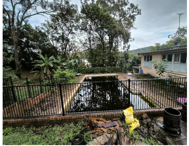
Figure 24 – 163 A Darley St backyard pool.
