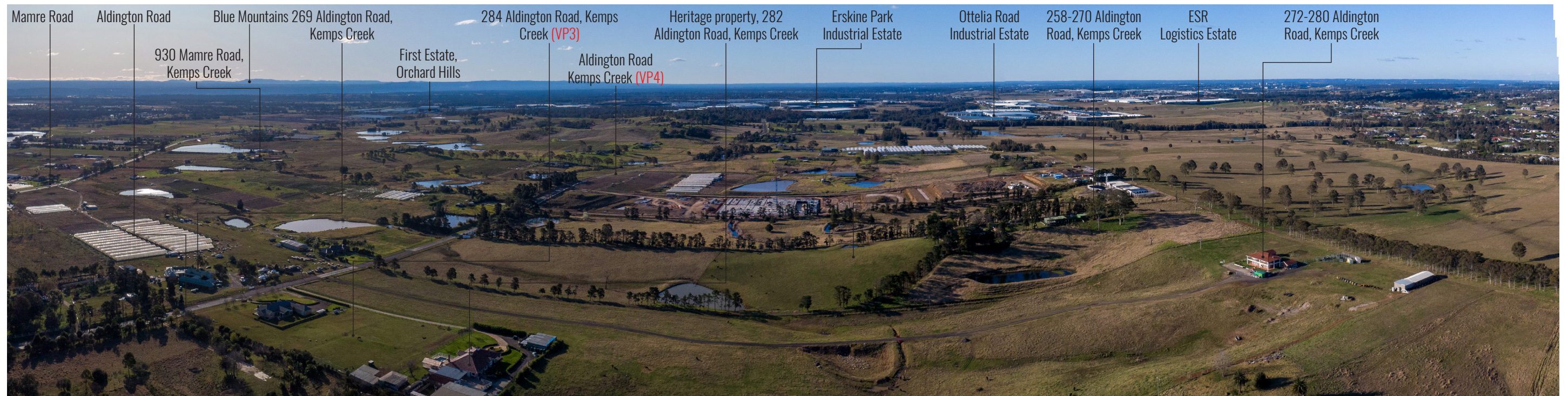
Figure 11: Drone at Position 2 - 120m AGL looking North
