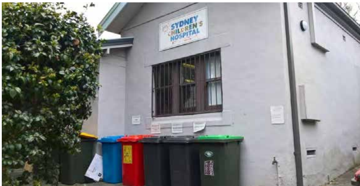
Photo 35 - Eurimbla Avenue Properties - domestic paints and building materials
