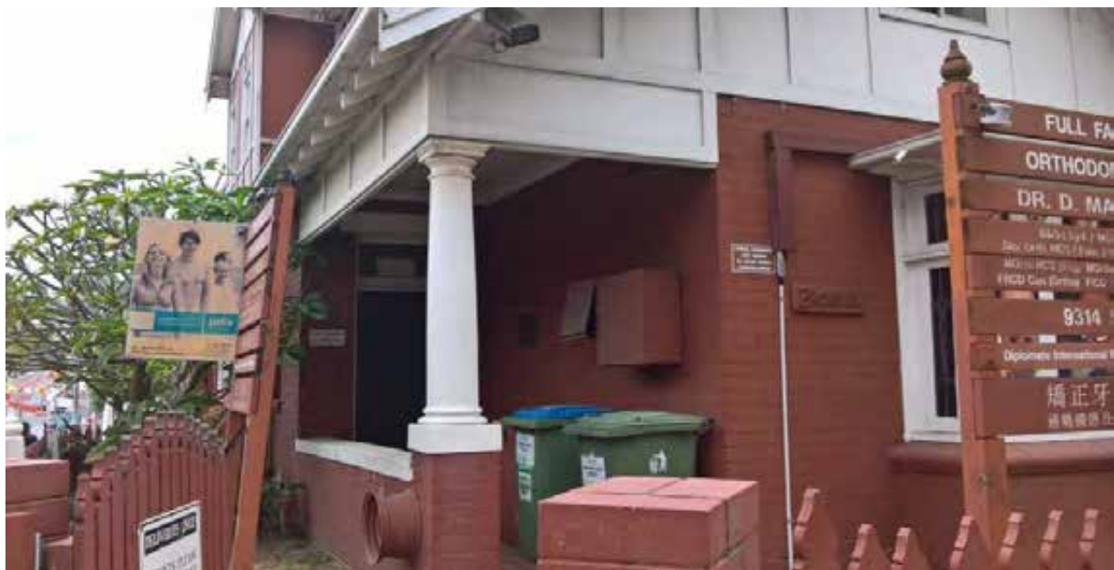
Photo 18 - Corner of Botany and High Street - commerical property
