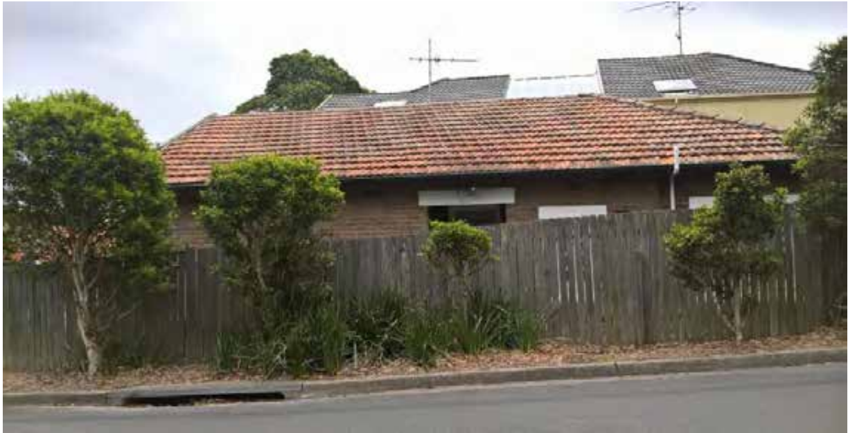
Photo 39 - Hospital Road (rear of properties on Magill Street)
