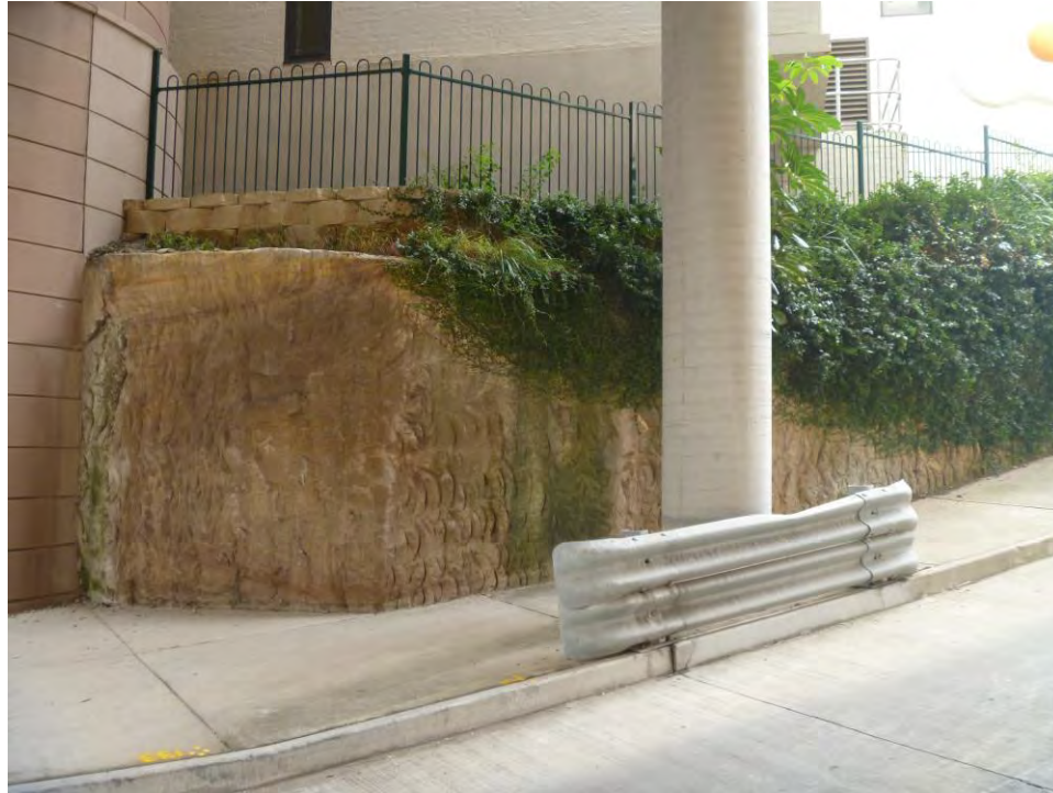
Photo 3 – Medium to high strength sandstone cutting, up to 2 m high.
