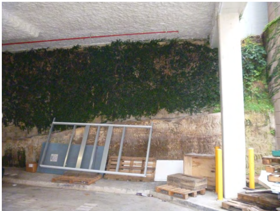
Photo 4 – Medium to high strength sandstone cutting, up to 2 m high.
