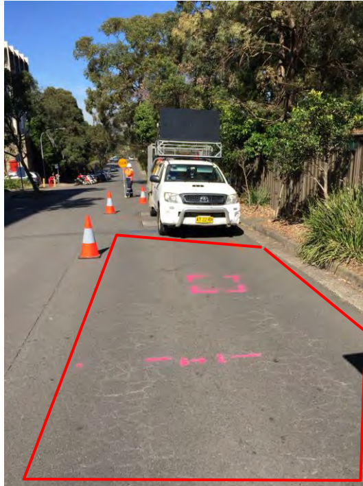
Photo 5 – Crocodile cracking along wheel paths in Hospital Road north-bound (near borehole BH2).
