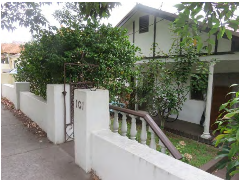
Figure 5.7: View looking northeast showing prominent drop in ground level within 101 Botany Street property on the corner of Magill Street.
