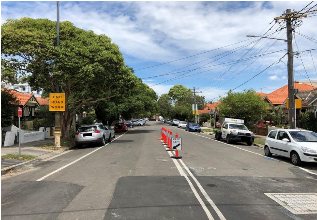
Figure 2-6 Eurimbla Avenue; looking south (Source: Advisian, 2017).
