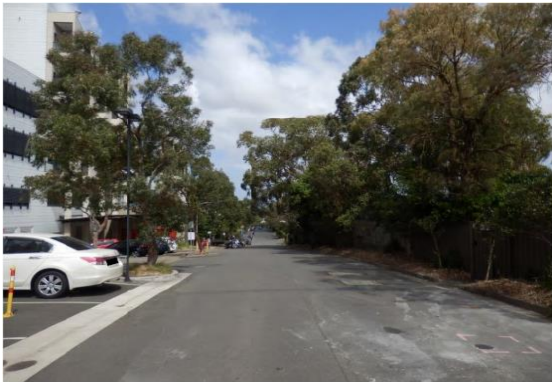
Figure 2-13 Hospital Road; looking south from Ainsworth Building (Source: Advisian, 2017).
