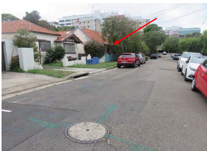
Figure 5.8: (Right) View looking east along public access corridor at rear of Magill Street. Modern stormwater service arrowed.
