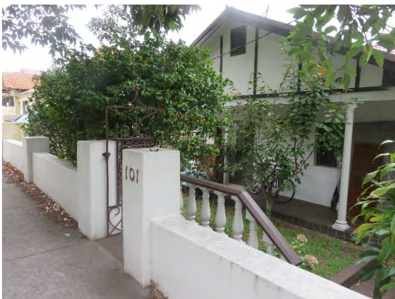
Figure 5.6: View looking northeast showing prominent drop in ground level within 101 Botany Street property on the corner of Magill Street.
