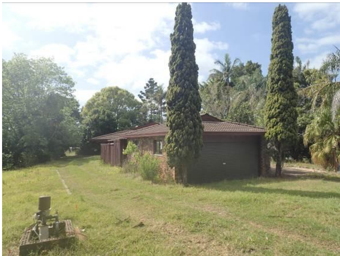
Plate 8 – Example of one the existing single story dwelling to be demolished, located within the Project alignment adjacent to the west of the proposed compound site.
