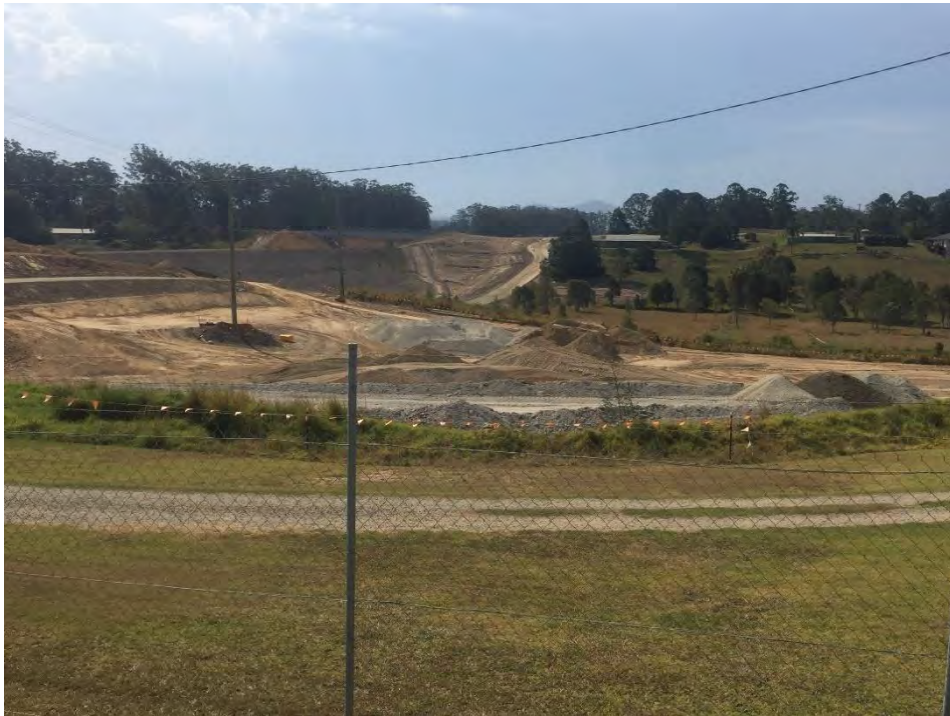
Photo 1: Looking Towards North West From Hillslope Over Proposed Car Park Area
