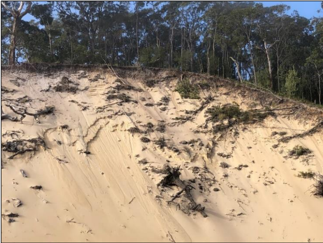
Plate 1: Example of unstable angle of repose on existing landform to be intersected with 20° batter.
