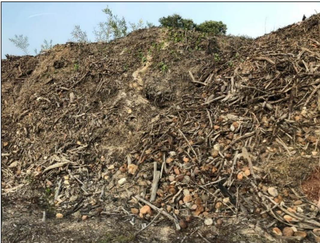
Plate 2: Example of using coarse material as protective cover to stockpile onsite.
