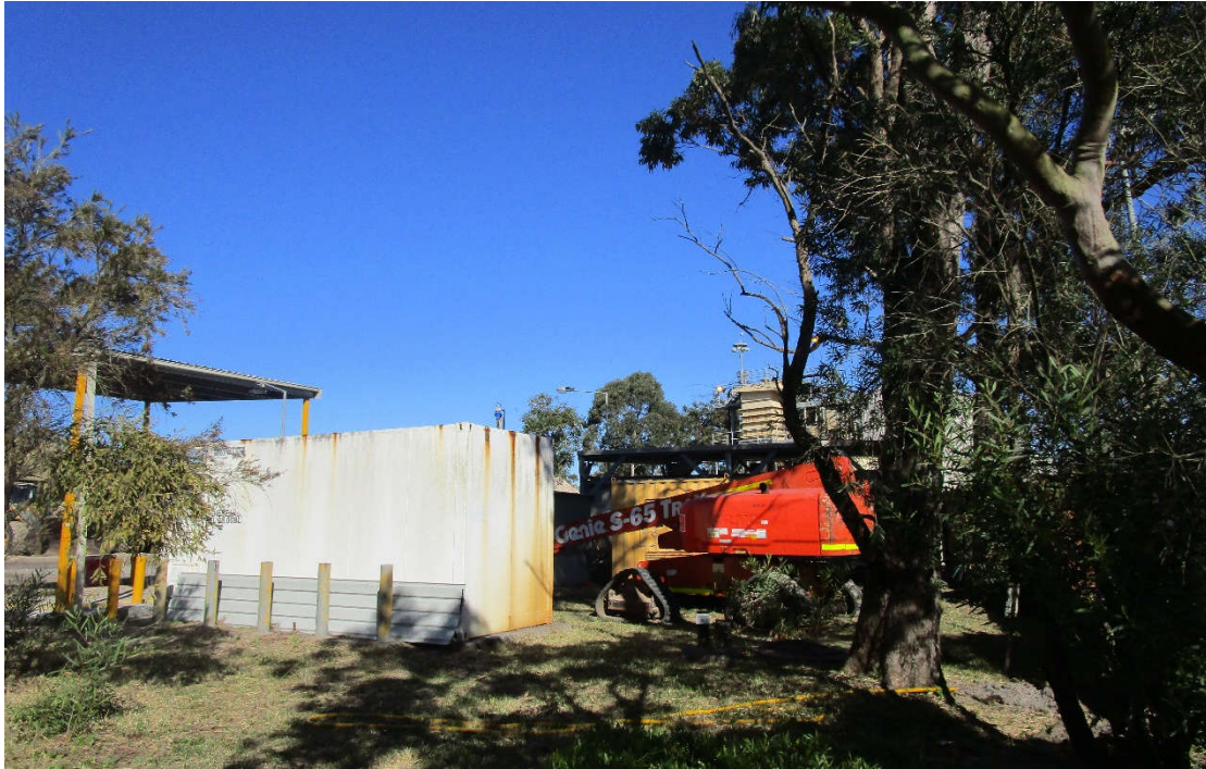
PHOTOGRAPH 3 – DIESEL FUEL STORE
