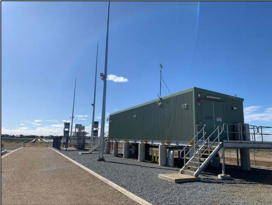
Plate 5: View of site infrastructure showing bushland colour palette for buildings. To reduce potential glare and light-spill issues, non-reflective construction materials were utilised and lighting is used on an as-needed basis, rather than being automatically activated at night.
