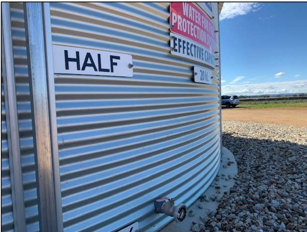
Plate 6: View of the 20,000L on-site firefighting water tank fitted with a 65mm Storz type valve in accordance with Development Consent Schedule 3, Condition 25(b).
