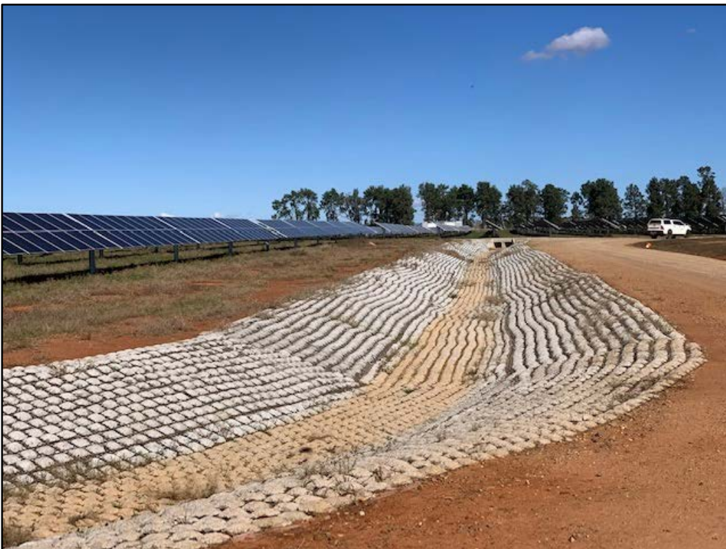
Plate 8: View of the stabilised drainage channel adjacent to the internal access road. This structure was designed and constructed to ensure unimpeded passage of water through the site and reduce the potential for erosion and/or sedimentation impacts.
