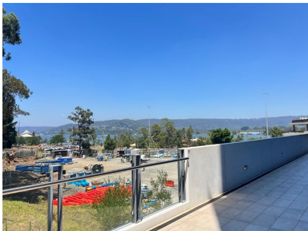
Picture 1 View of site from 32 Mann St, looking south
