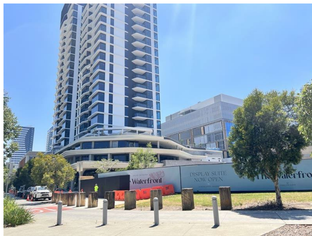
Picture 4 View of the site from Gosford Waterfront Park, looking northeast
