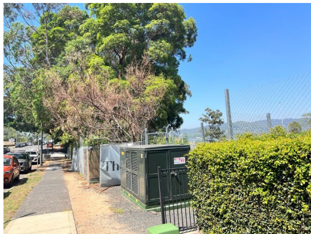
Picture 2 View of the site from Mann St, looking south
