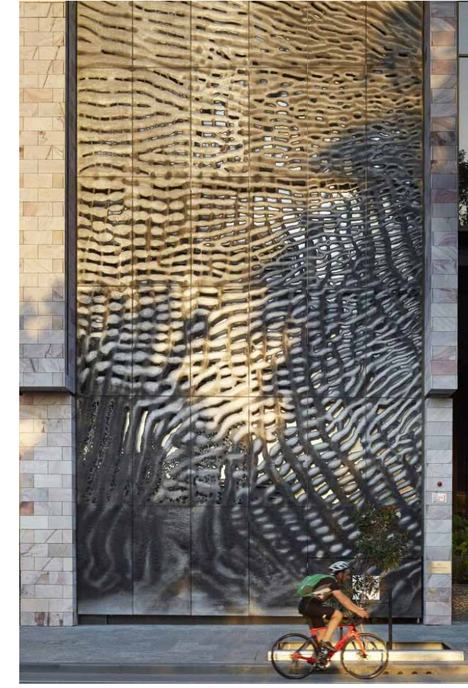
Catherine Woo, Cascade , 2020. The shimmering material replicates the movement of water, fabricated in recycled cast aluminum over the facade. The artist harnesses light with the reflective surface, showcasing the transient texture of place onto physical material. Photo: UAP Robert Frith Acorn Photo
