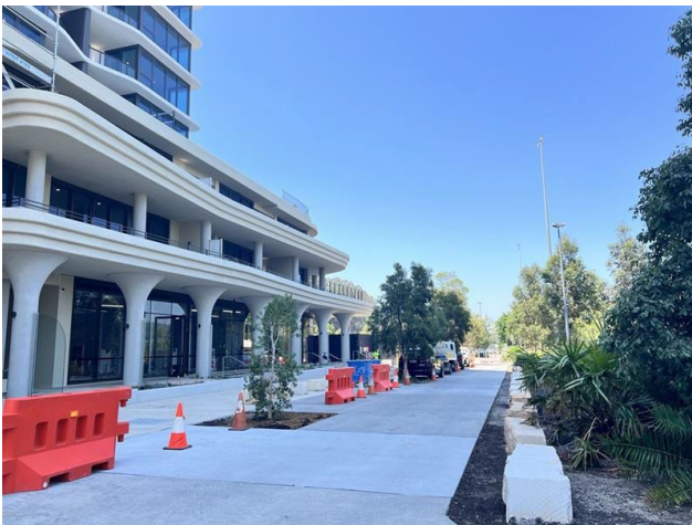
Picture 5 View of northern tower from Baker St, looking south
