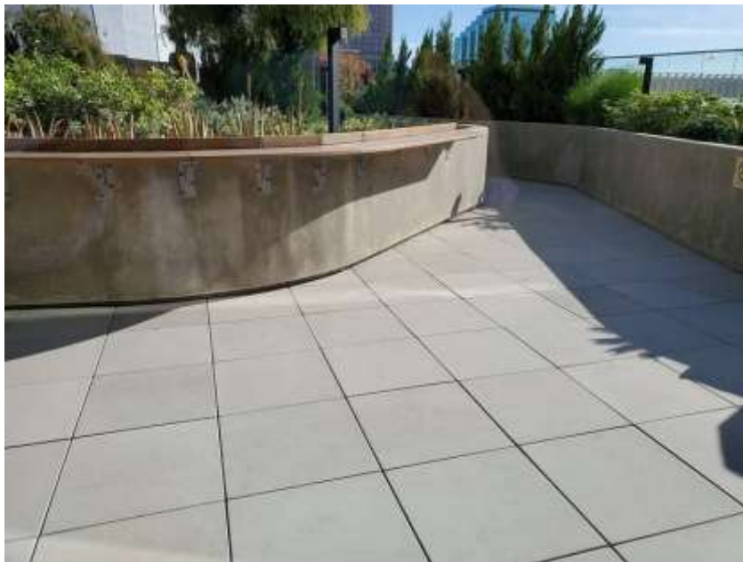
Figure 9 Roof Terrace Pavements with High SRI Materials
