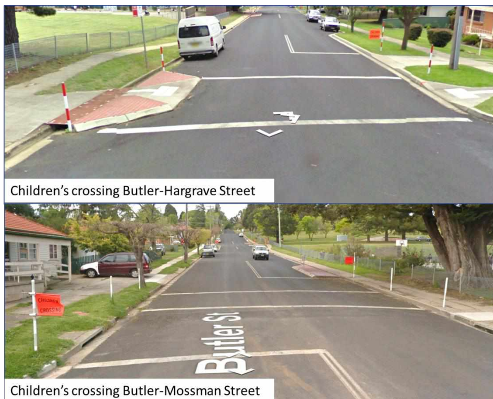
Figure 2-8: Children's crossing across Butler Street
