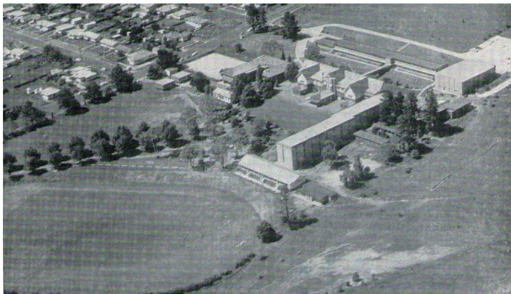
Figure 6 – Oblique aerial of Armidale High School, 1969. (Source: The Armidale of Yesteryear Facebook page, 19274988_1330255717021848_4728667350417455756_n)
