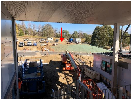
Figure 15– View from the walkway located within Zone 3 and Zone 4, towards the location for the proposed new Multi-Purpose Hall, indicated by the red arrow. NBR SARCHITECTURE, 2020.
