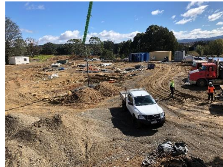
Figure 16– Photograph of the the location for the proposed new Multi-Purpose Hall. NBR SARCHITECTURE, 2020.
