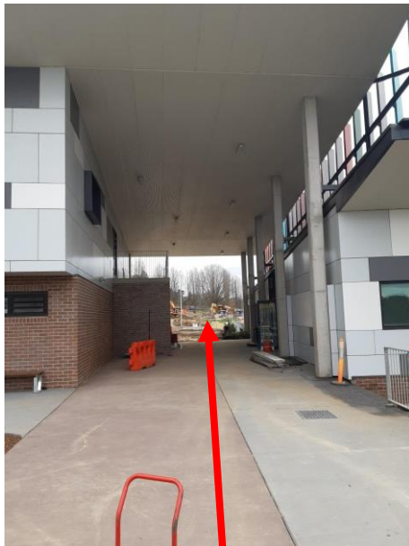
Figure 13– View from B-Block, along an existing pathway, looking south towards the location for the proposed new Multi-Purpose Hall. (NBRSARCHITECTURE, 2020)
