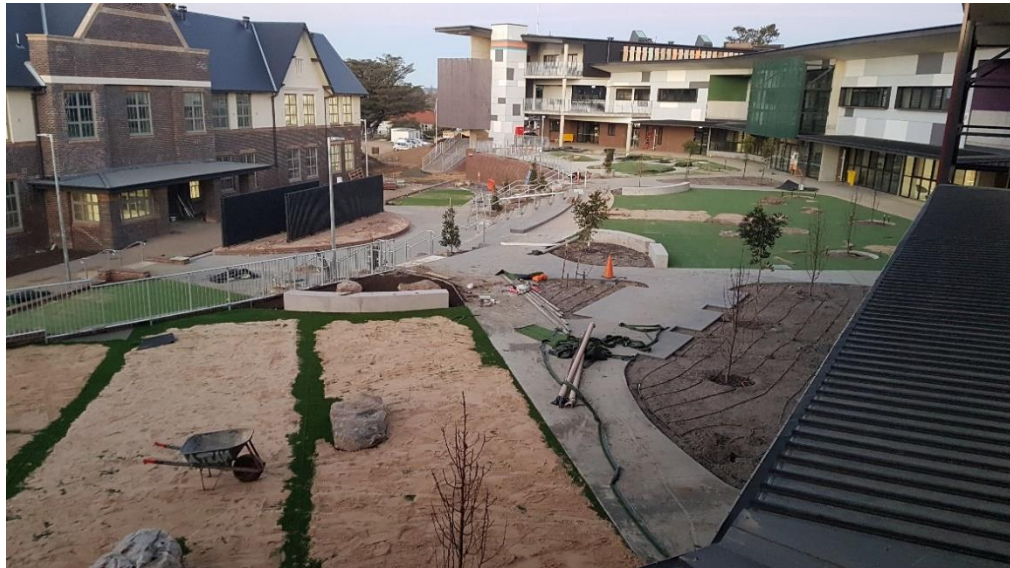
Figure 10 - View of new classroom block looking east towards administration area. B Block located to left of photograph. (NBRSEARCHITECTURE, 2020)
