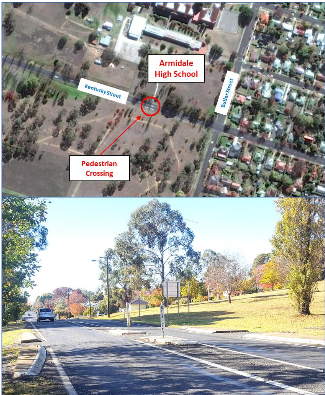
Figure 2-10: Pedestrian crossing across Kentucky Street
