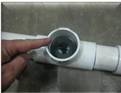
Figure 8. Install Flow Discs.
