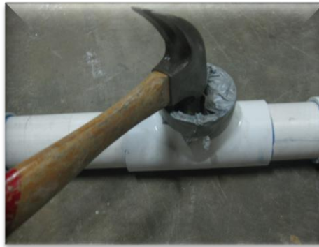
Figure 7. Exposing Holes in PVC Fittings.
