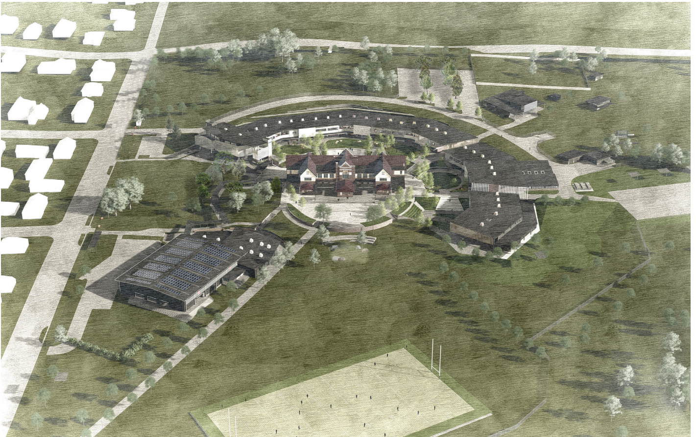
VIEW FROM MANN STREET
