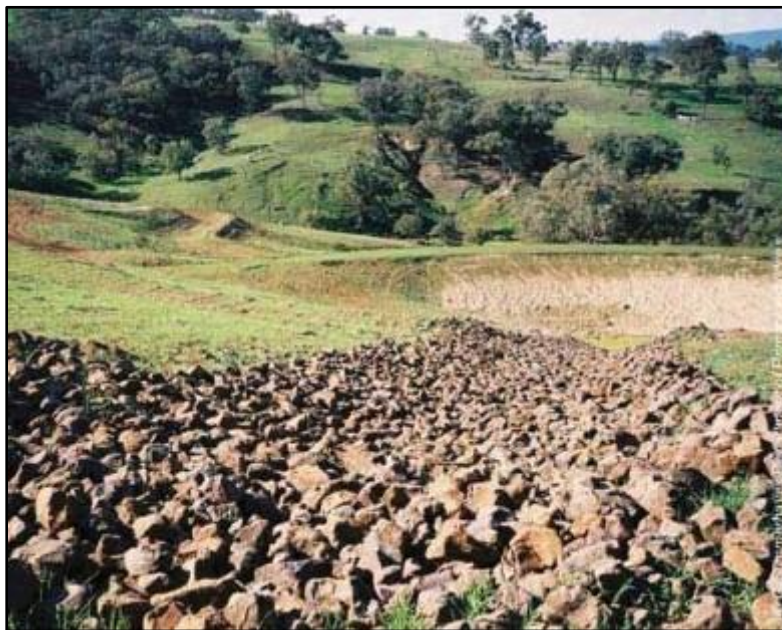
Figure 4: Rip-rap rock waterways conveying runoff to a sediment basin
