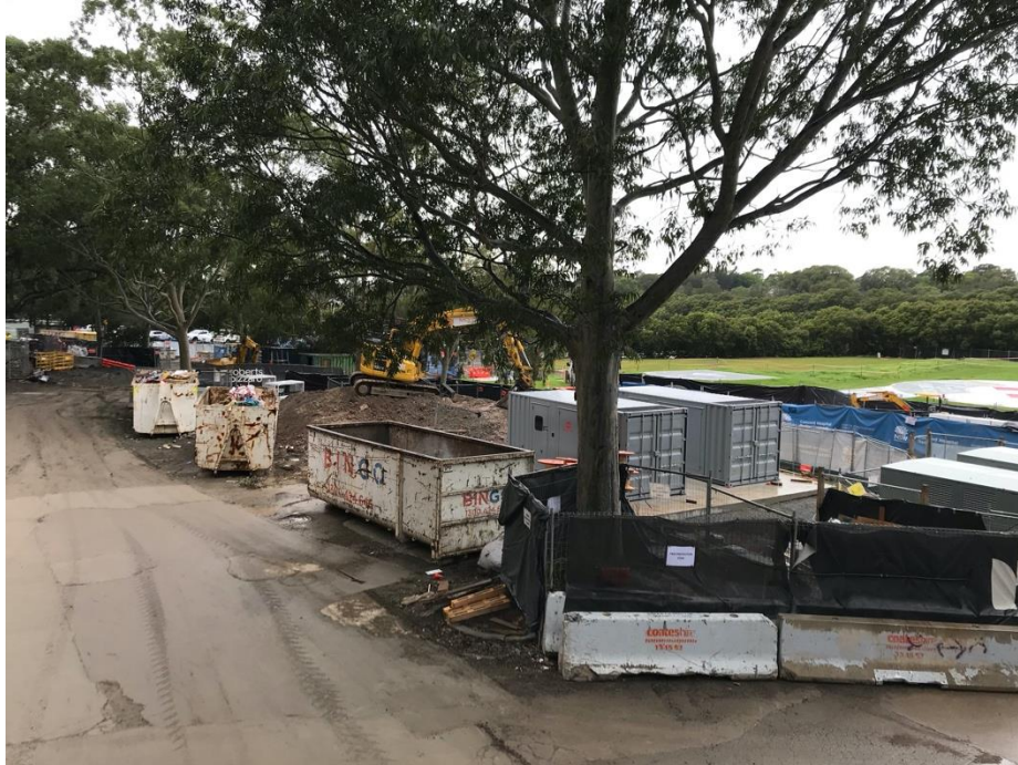
Photo 3 – Waste bins available and tree protection installed for protected trees.
