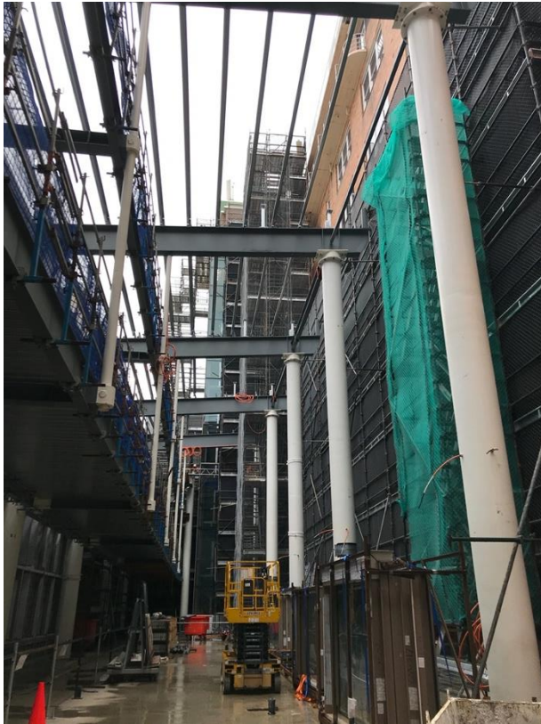
Photo 5 – Steel works in the Atrium area connecting the existing hospital with the new development.
