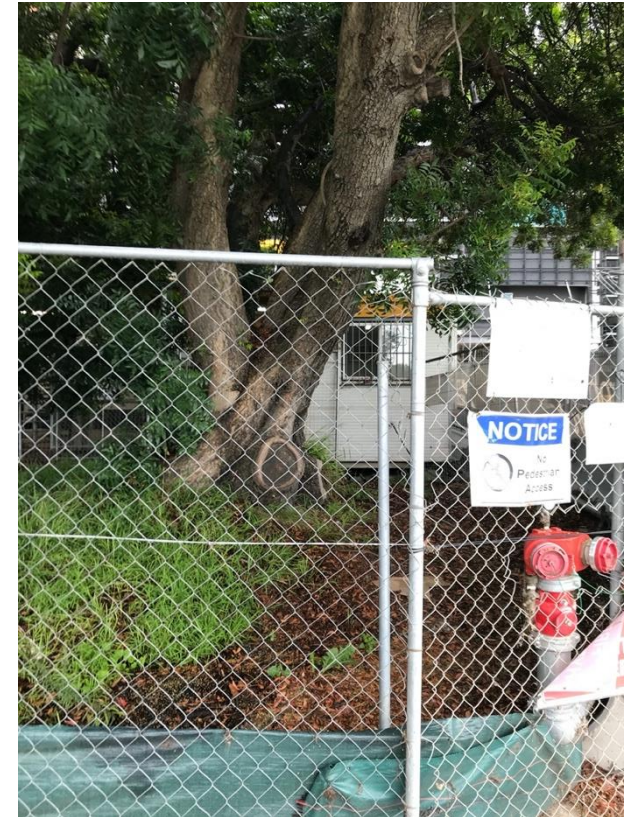
Photo 4 – Tree protection and silt fence installed.
