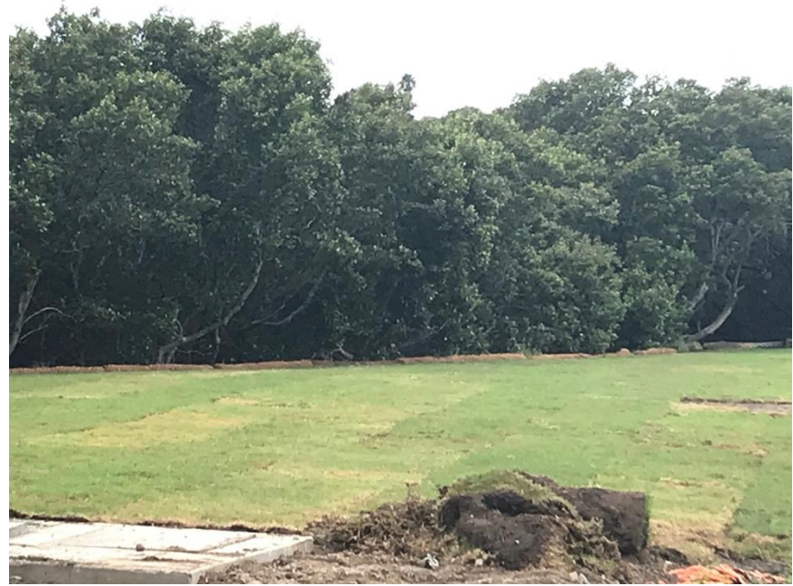
Photo 6 – Coir logs in the perimeter of the site during turf installation in the helipad area.
