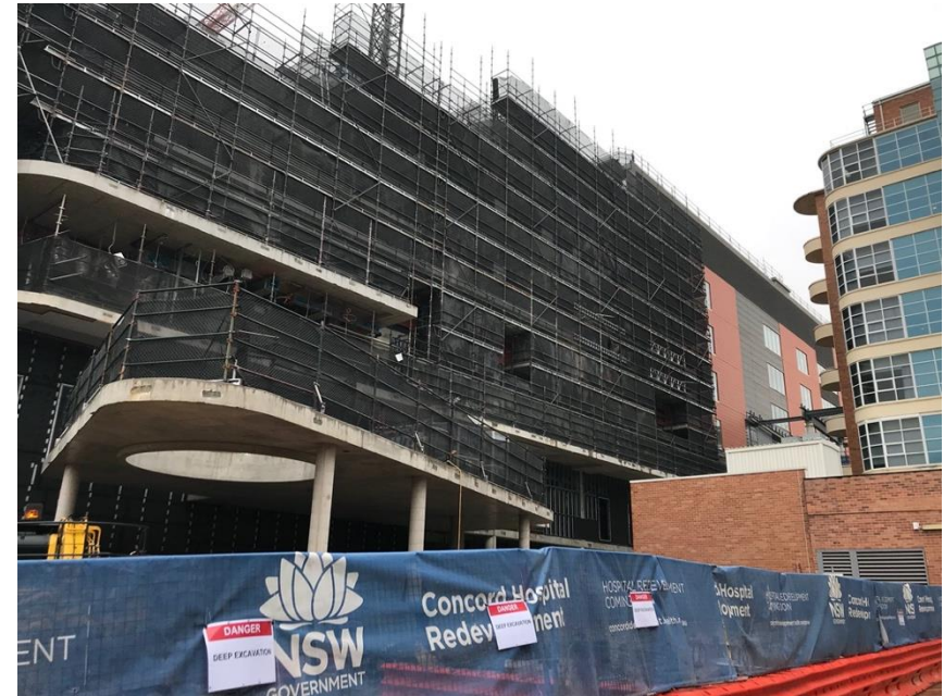
Photo 2 – Works progressing in a future hospital entrance, adjacent to the old hospital building.
