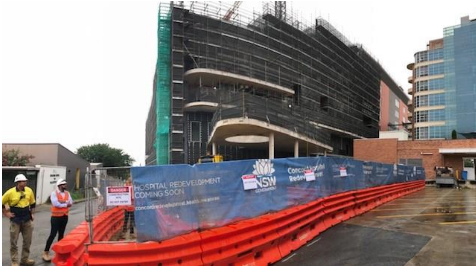
Photo 13 – Looking at the future emergency entry of the new building.
