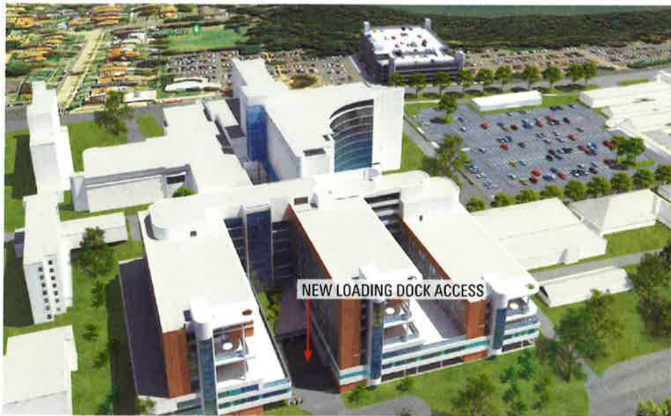
View from Site. Stage 1 in the foreground.
