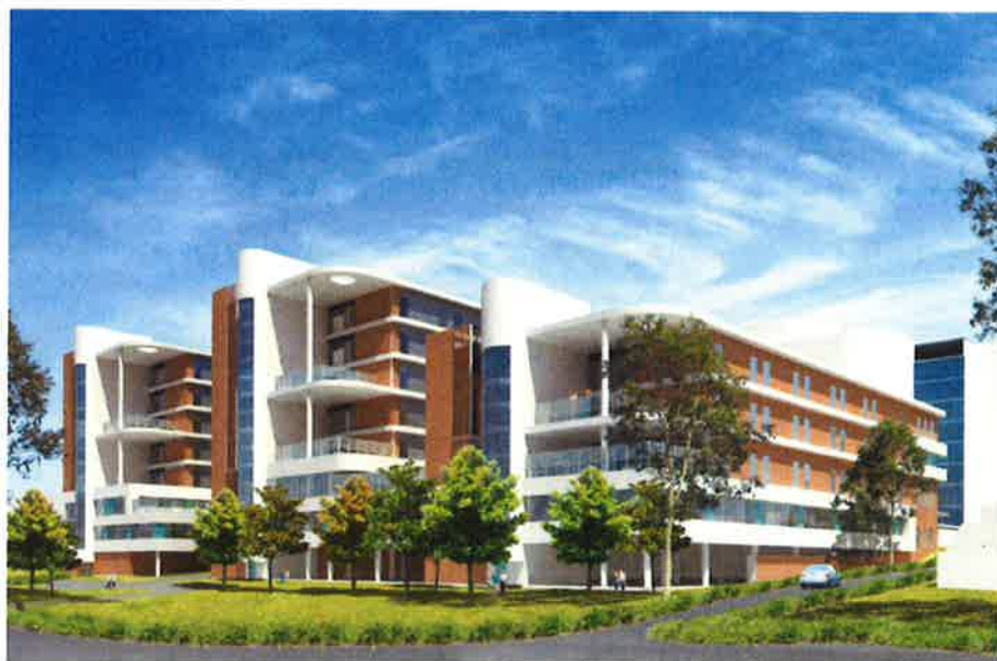
Street level view of new Stage 1.
