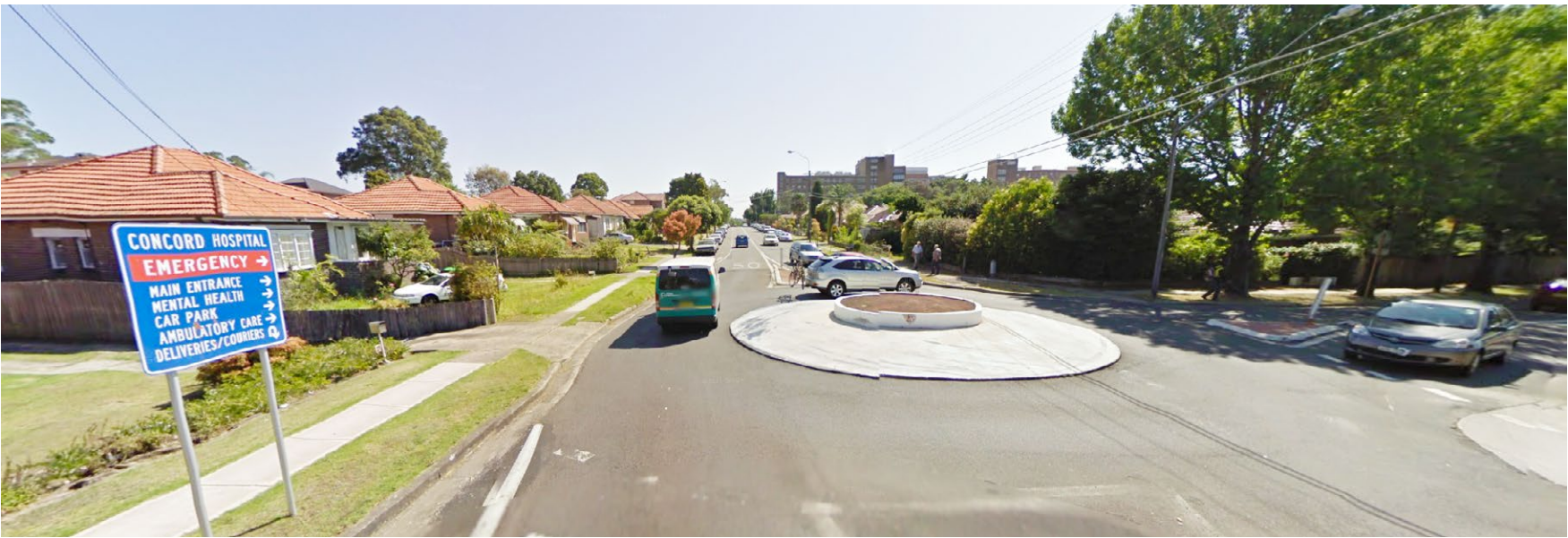
Corner Hospital Road / Nullawarra Avenue. Directional sign is parallel with main traffic and not visible from the required distance
