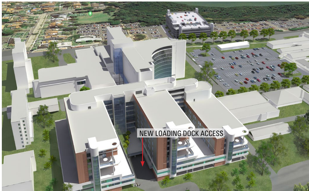
View from Site. Stage 1 in the foreground.
