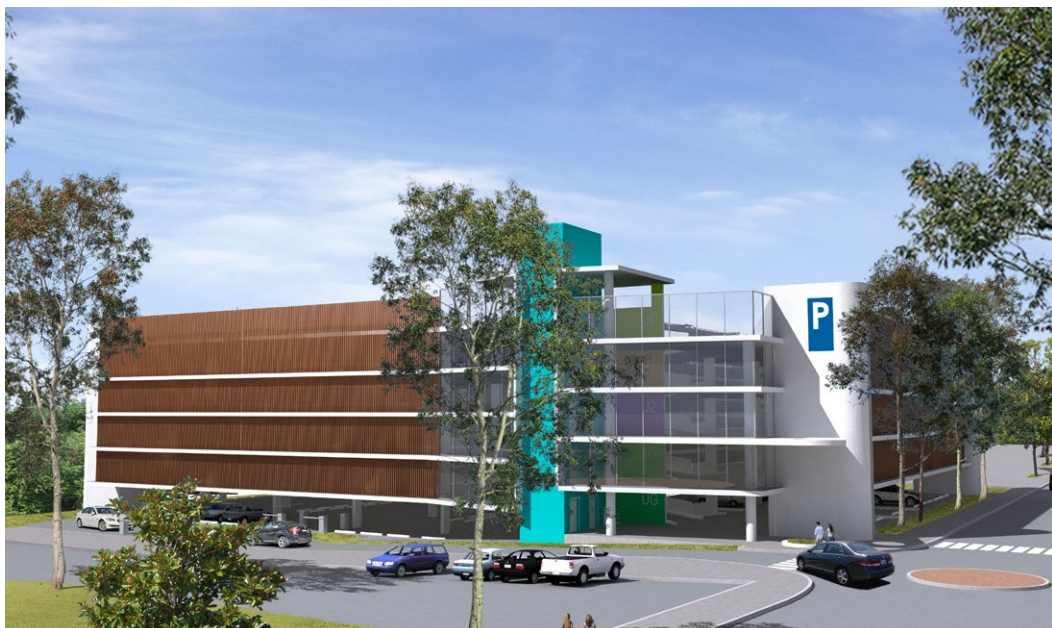
New multistorey carpark.
