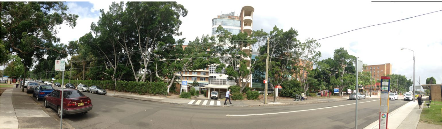
View of the Main Building from across Hospital Road
