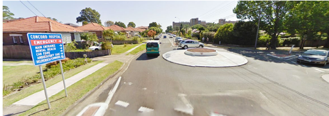
1. Corner Hospital Road / Nullawarra Avenue Directional sign is parallel with main traffic and not visible from the required distance
