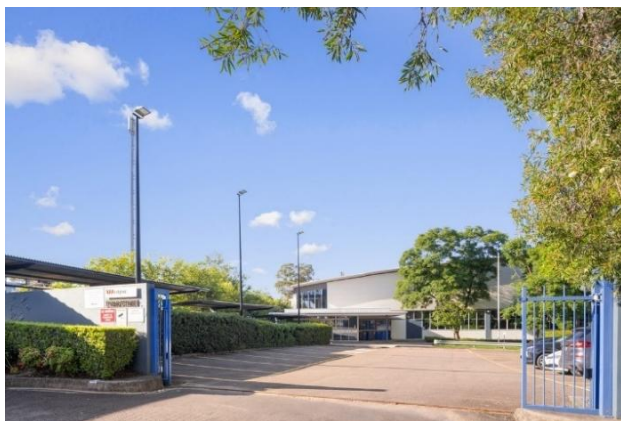
Figure 3 Entrance to Building Carpark
