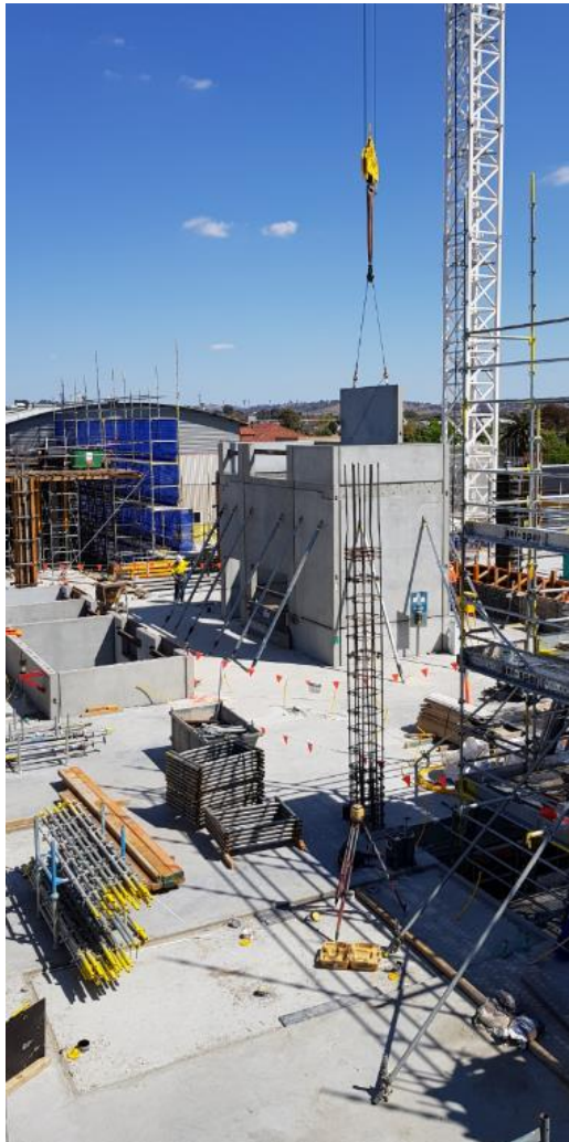
Figure 7 Precast concrete panel installation & slab construction for level 1 Suspended Slab
