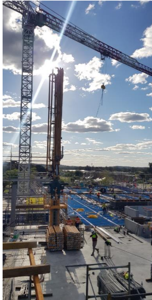
Figure 7 Precast concrete panel installation & slab construction for level 1 Suspended Slab
