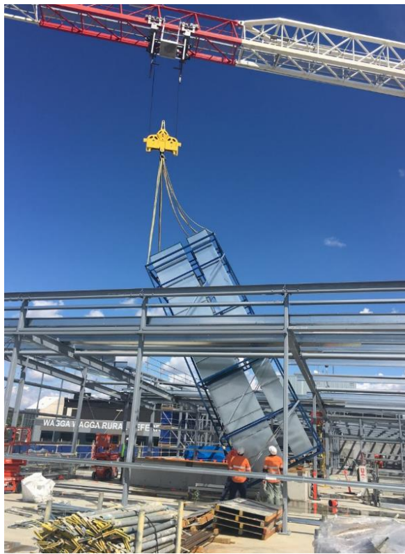
Figure 6 Prefabricated Module Installation
