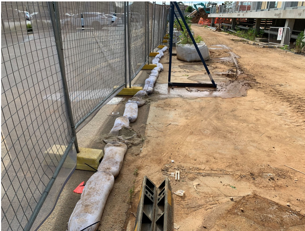
Sediment control at pit
