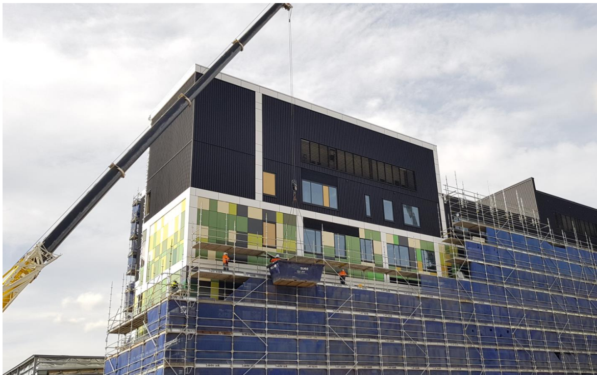
Figure 6: Façade installation and removal of perimeter scaffold
