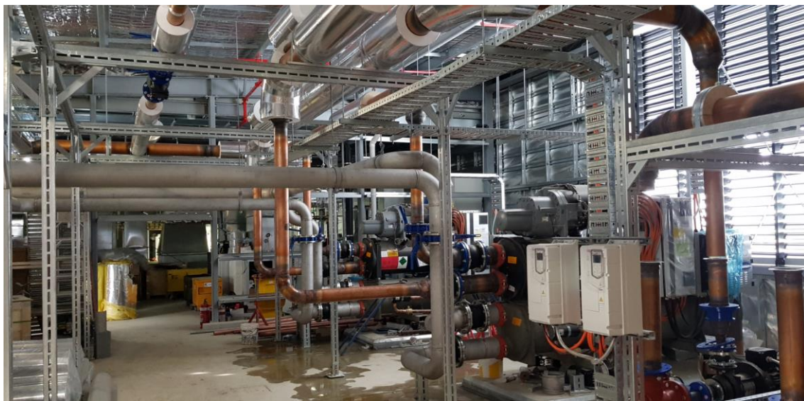
Figure &: Plant Room Works – Chiller Plant shown above
