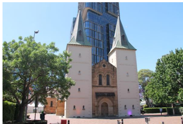
Figure 40. View of St John's Anglican Cathedral (SHR no. 01805) facing southeast in the direction of the study area
