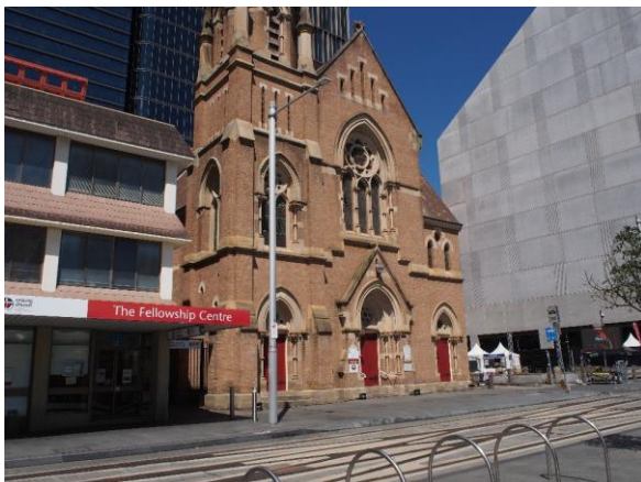
Figure 37. View of Leigh Memorial Church (LEP no. I586), northwest of the study area, facing southwest
