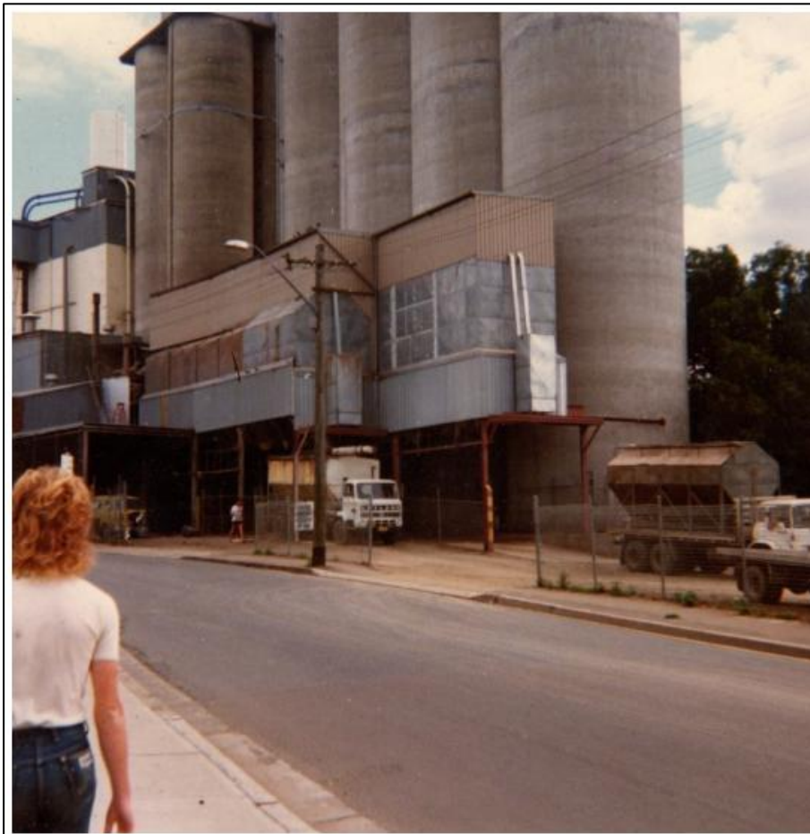
Figure 12. Photograph of the mill's stockfeed outloading bins, with four 1000 ton concrete silos behind (Source: John McCorquodale, 2021)
