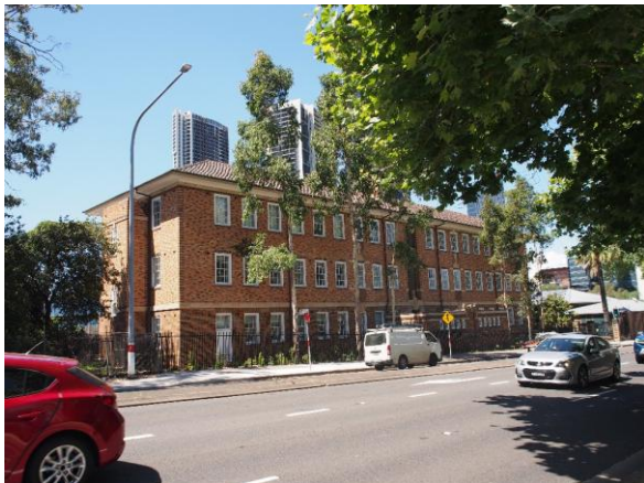
Figure 49. View of the former Kings School group (SHR no. 00771) in the direction of the study area, facing southeast on O'Connell St
