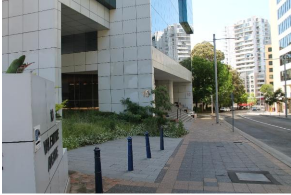
Figure 23. View of the extant buildings occupying the study area, facing southeast on Valentine Ave
