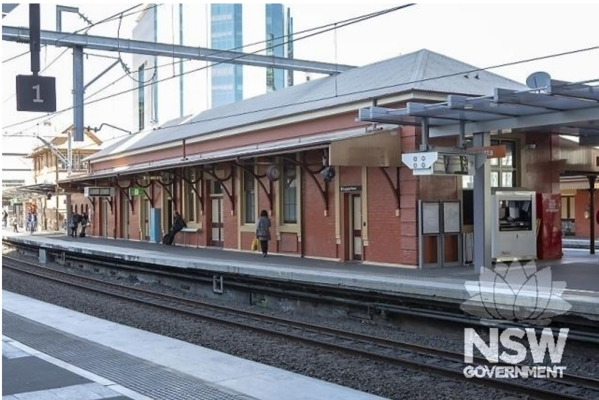
Figure 66: View of the historic platforms at Parramatta Station 39
