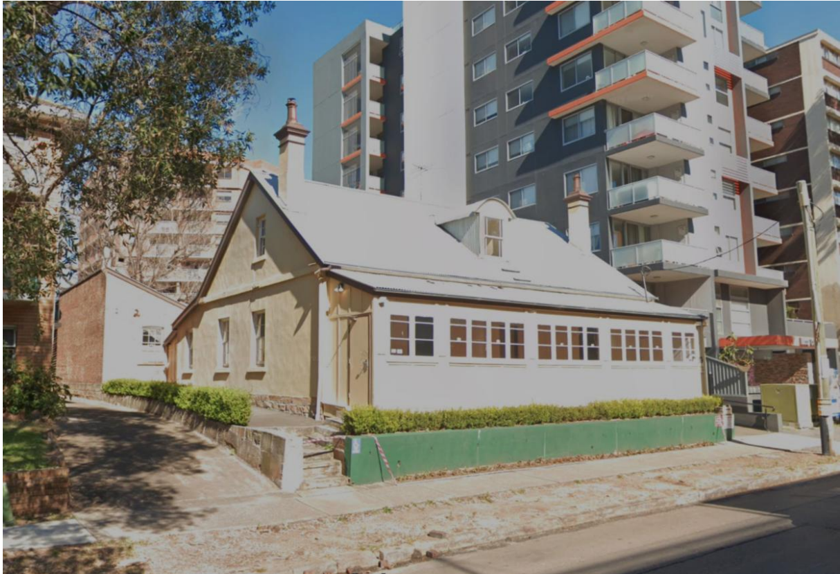
Figure 71: Lennox House (Source: Google Streetview, 2023)
