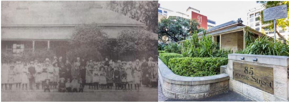
Figure 73: Image showing Perth House used as a school in 1889 and a contemporary image of the building 54
