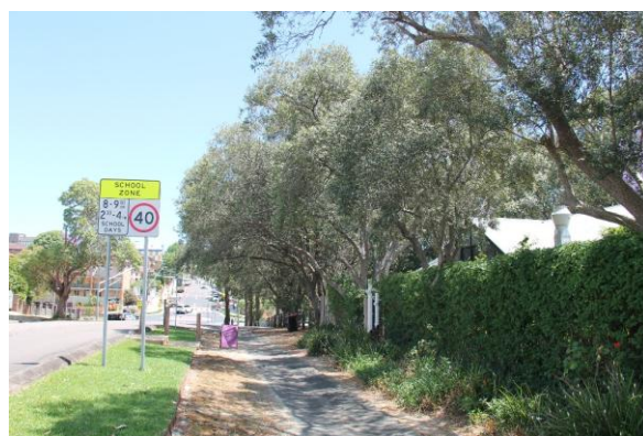
Figure 56. View of the southern boundary of Elizabeth Farm (SHR no. 00285) east of the study area, facing west on Alice Street
