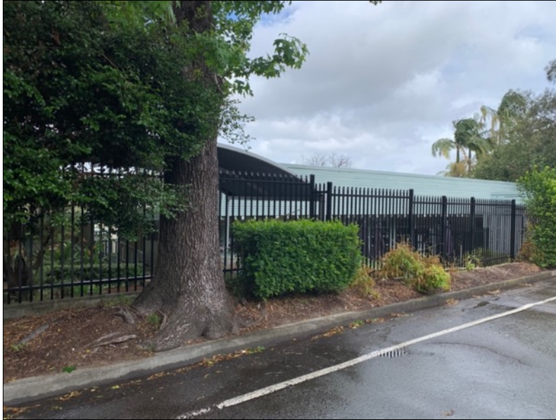
Figure 30: The Community Centre form the adjoining carpark.
