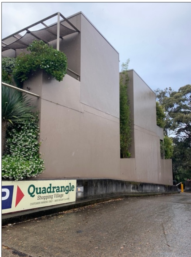
Figure 14: No. 116 Edinburgh Road as it presents to the site.
