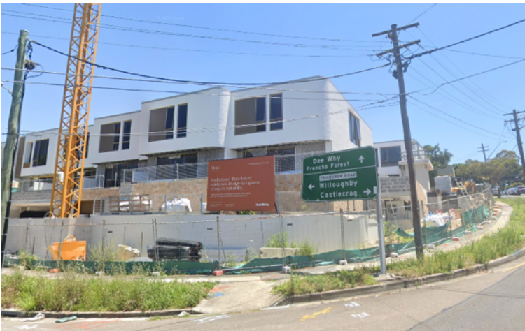
Figure 16: A recently completed , opposite the subject site, on the other side of Eastern Valley Way.
