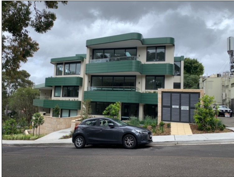
Figure 25: Recently completed flat building to the south of the Griffin Centre.
