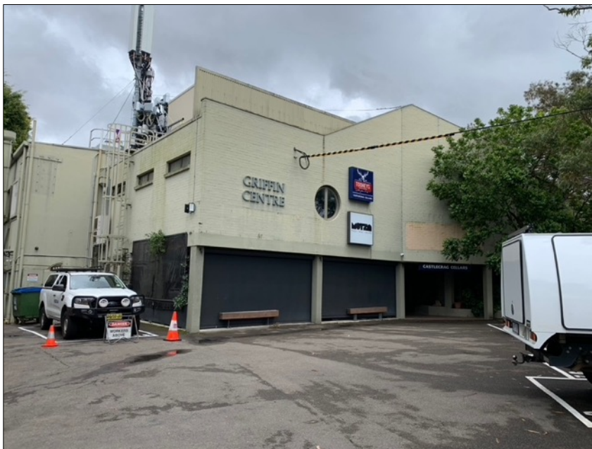
Figure 22: The side and rear elevation of the Griffin Centre.
