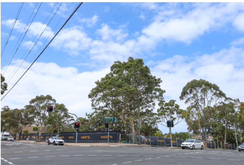
Figure 5: The site today with all buildings demolished.
