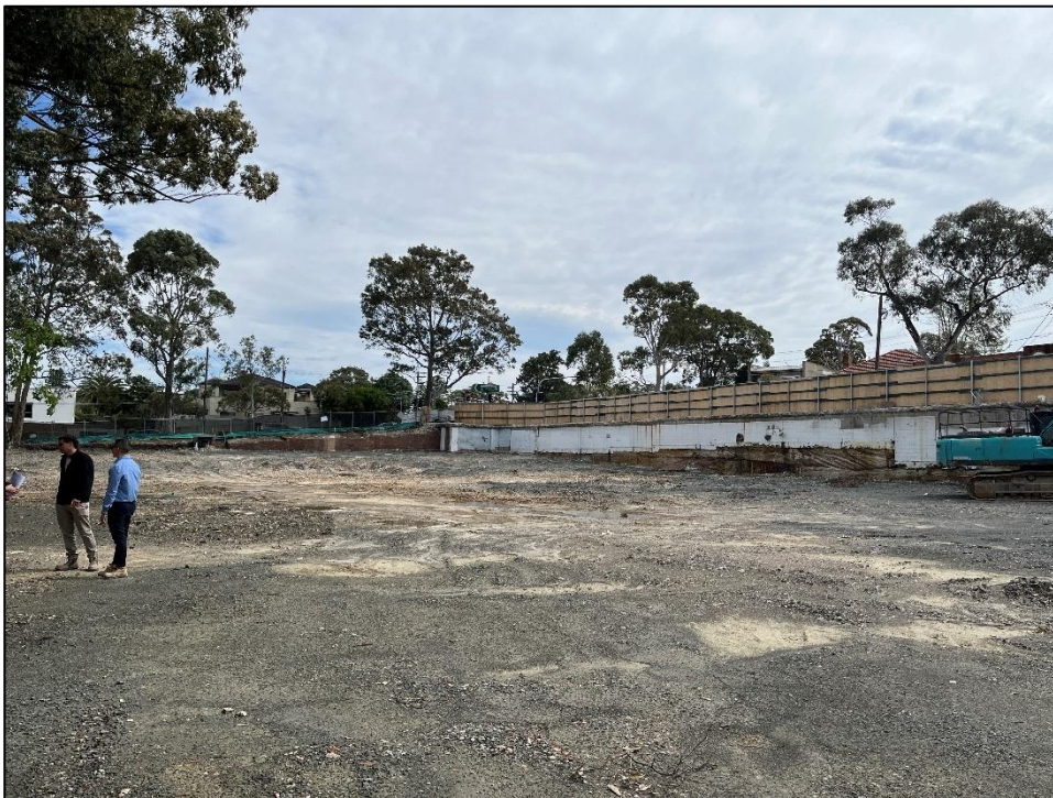
Figure 2 – Photo of existing site conditions, looking northwest, dated 17 September 2025
