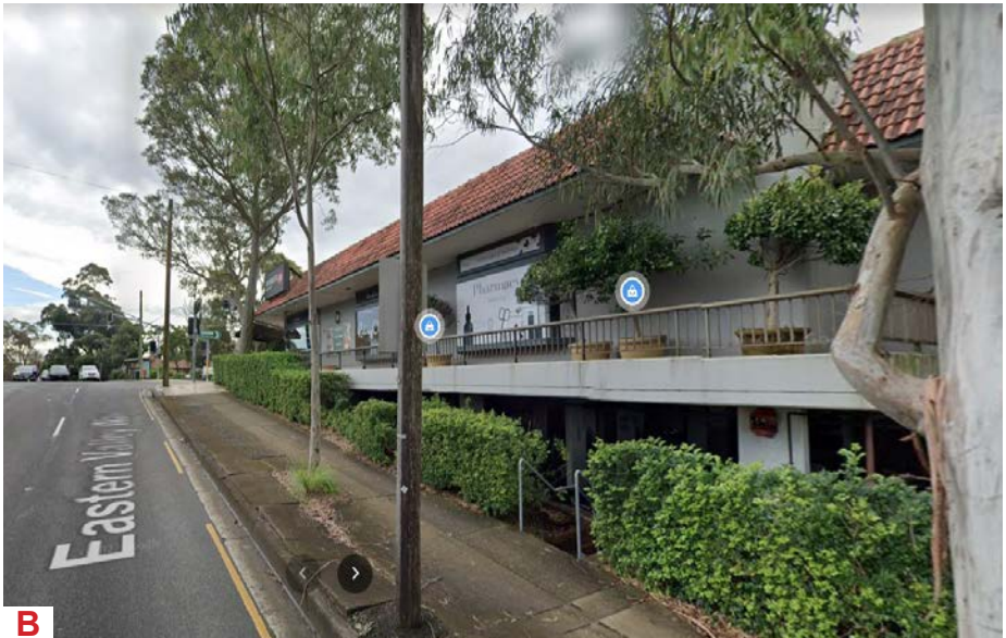
B View indicates how previous development was set down below street level to accommodate carparking
