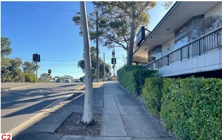
C2 Eastern Valley Way pavement condition.
