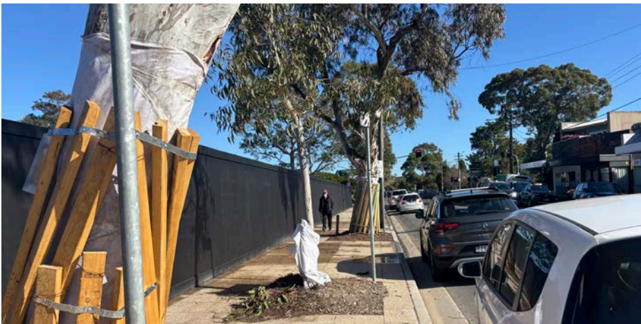
Tree protection along Edinburgh Rd and site hoardings
