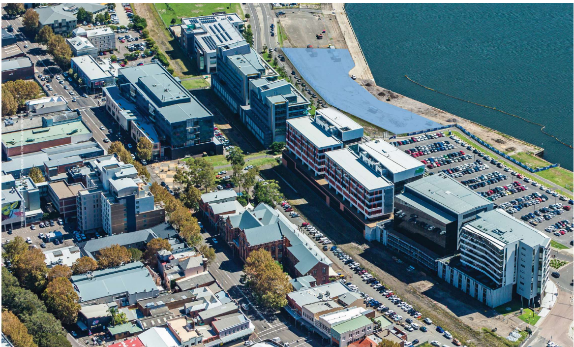
Photo above – Aerial image of the site in the emerging Honeysuckle precinct
