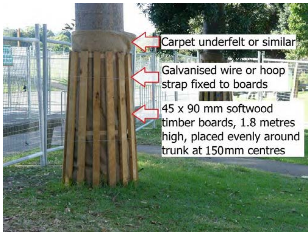
Figure 5 – Detail of Trunk Protection
