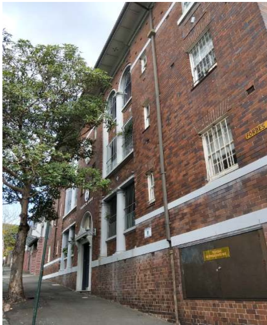
Photo 3 - Wilkinson House, used as the senior study centre, is one of the older buildings onsite.
