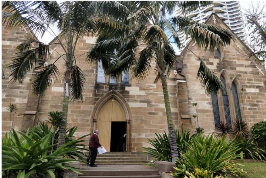
Photo 1 - Old church building repurposed in to the Great Hall, with garden beds out the front.
