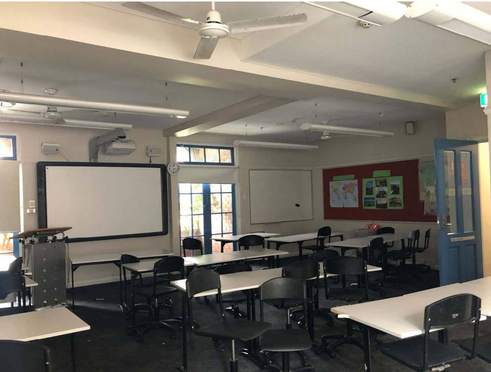
Typical classroom interior, showing location of former partition walls in ceiling.
