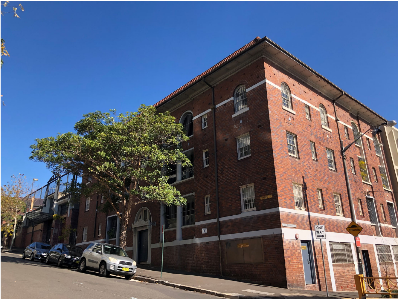
Wilkinson House, corner Forbes Street and St Peter’s Lane, Darlinghurst. Source: TKD Architects.
