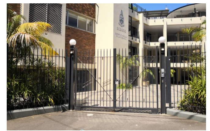
Bourke Street Gate
