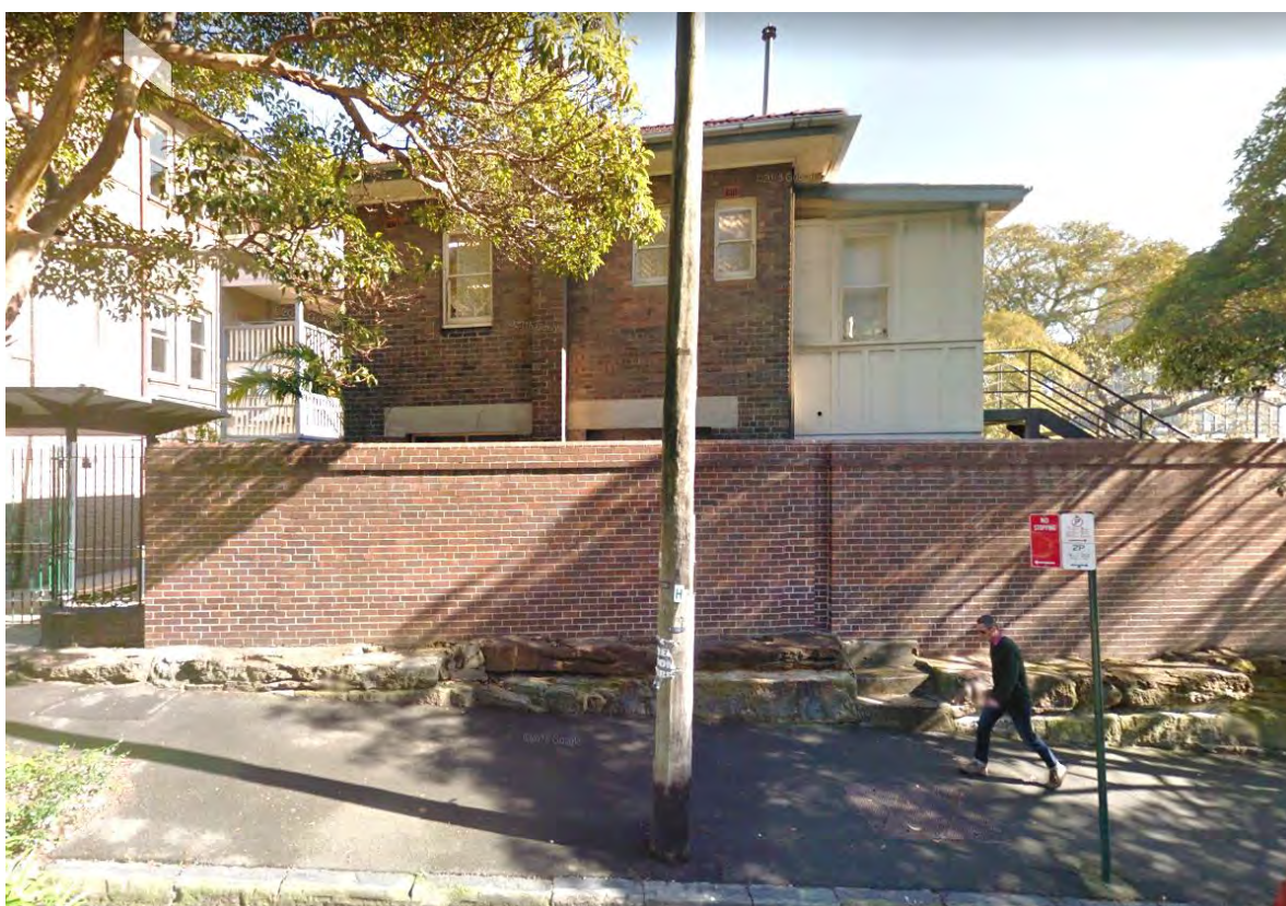
Figure 1.7: View northwards along Forbes Street showing bedrock exposed to the east of the Barham extension.
