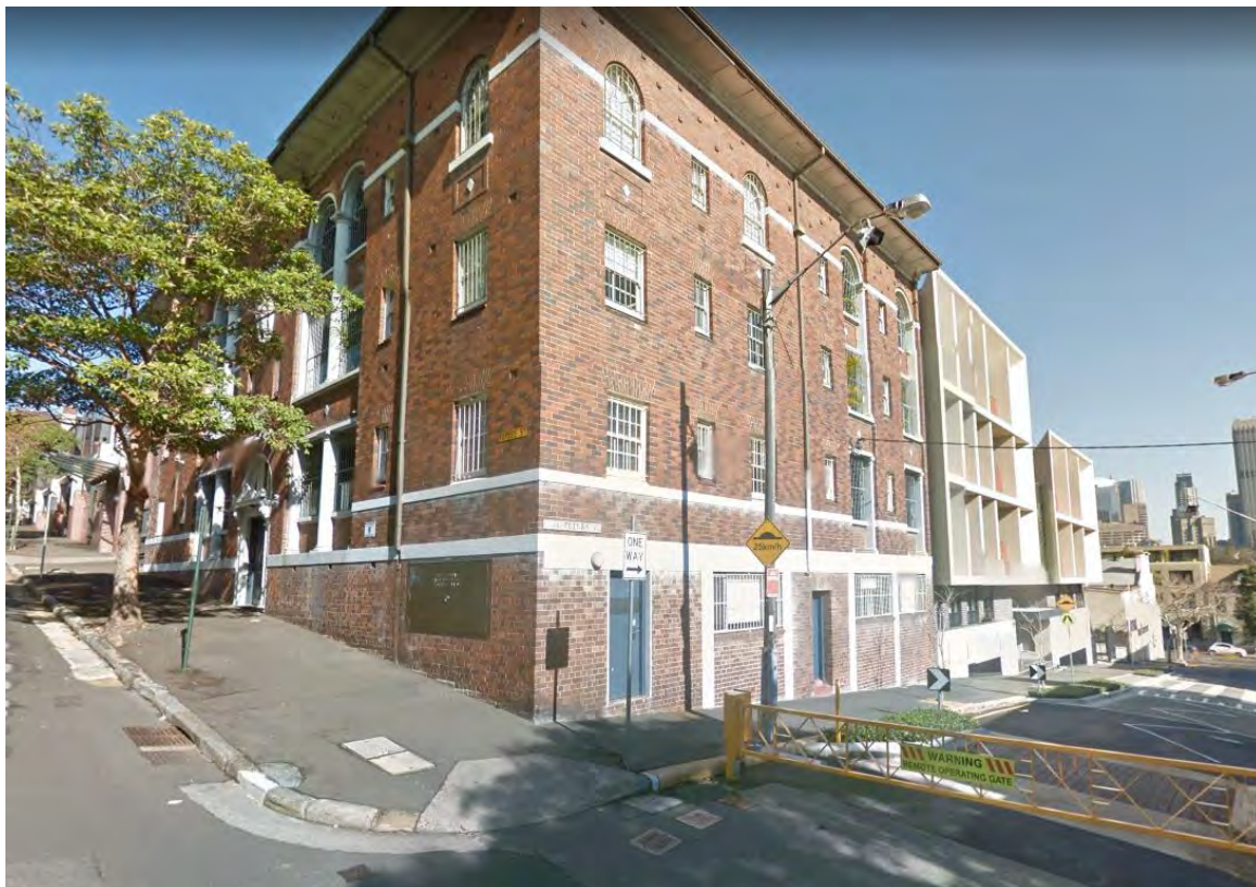
Figure 1.4: View southwest along St Peters Street showing Wilkinson Building cut into the slope.
